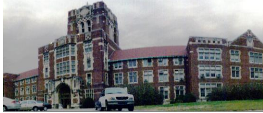
The Ayres Building from CCD camera
