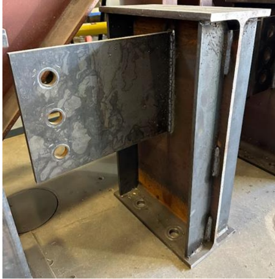
(a) Shear Tab Connection Plate
