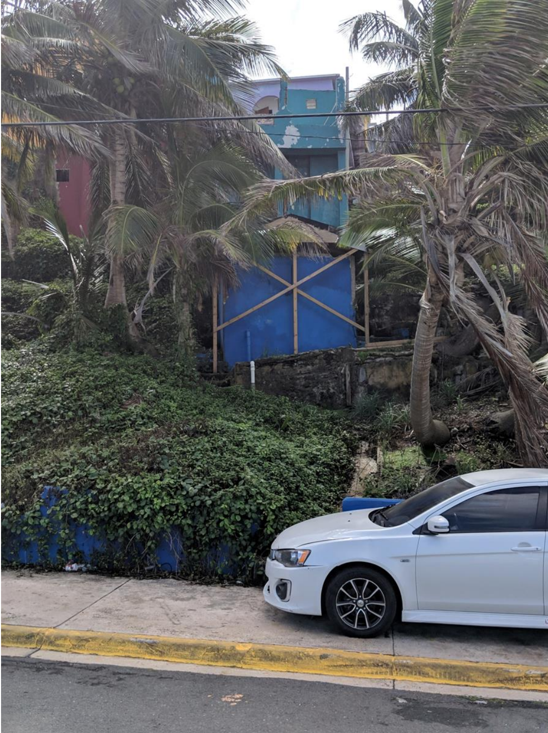
Figure 3.4 Tarp and Wood Frame Home
