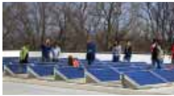
Figure 04: Sidwell Friends Solar roof (AIA Cote Top Ten, 2007)
