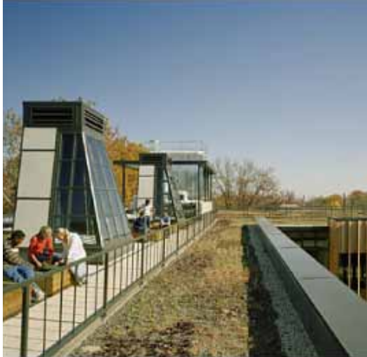
Figure 01: Rooftop view of Sidwell Friends School.
