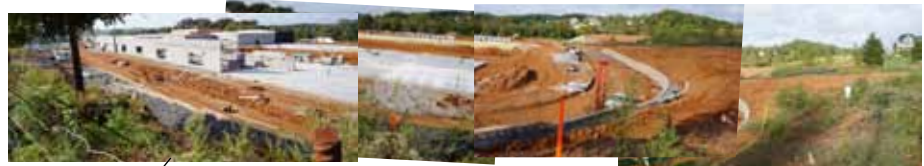
Figure 23: Photos from the site
