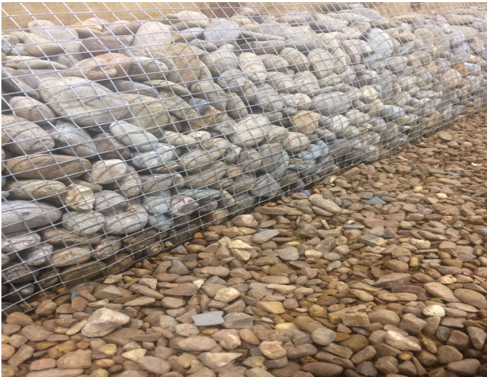
Figure 3.9. Gravel revetment with wire mesh support.
