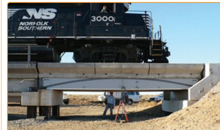
John Hillman stands below the 30-foot span of the first HCB-built bridge in Colorado while a locomotive pulls loaded cars across it.
