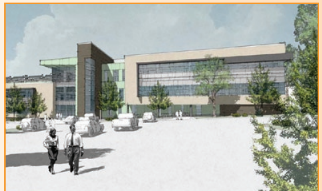
The Joint Institute for Advanced Materials (JIAM) facility
