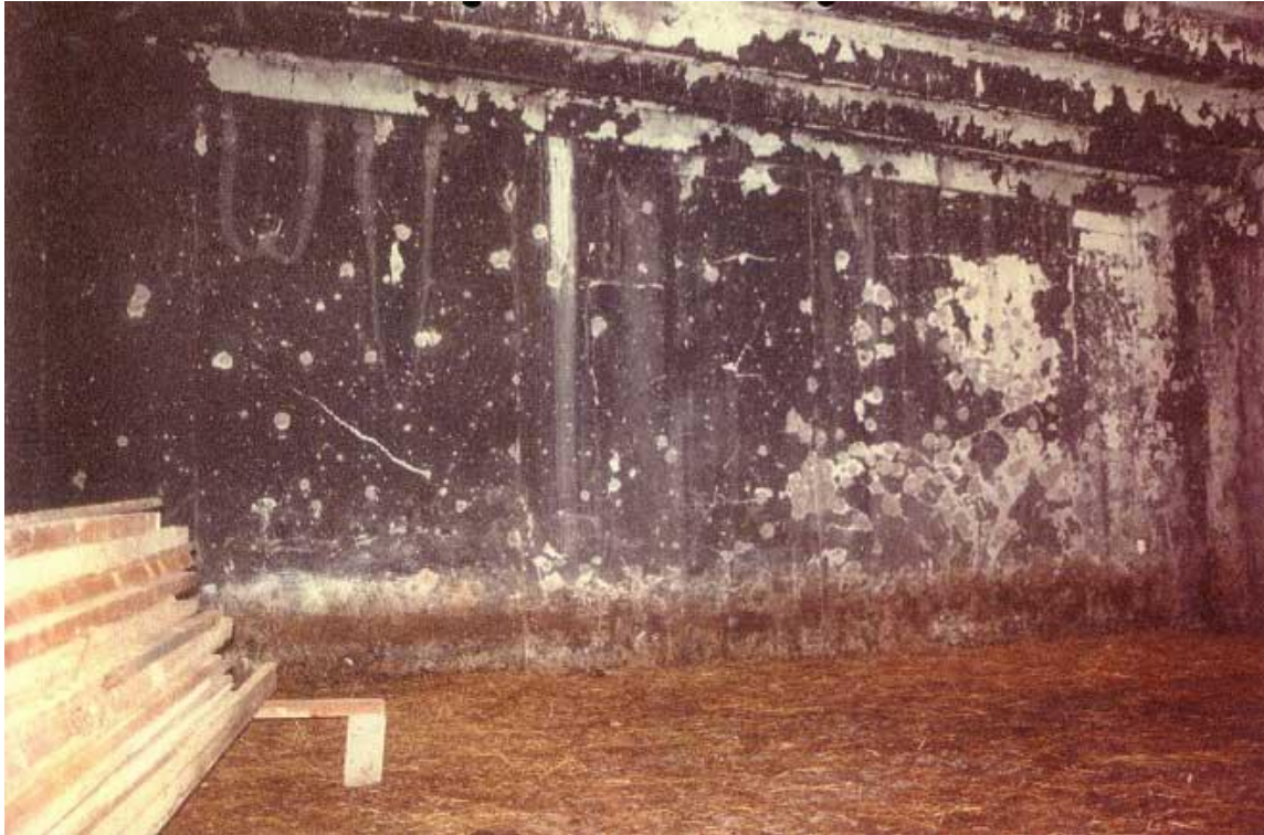
Figure 6. Interior of the Kravica warehouse.
