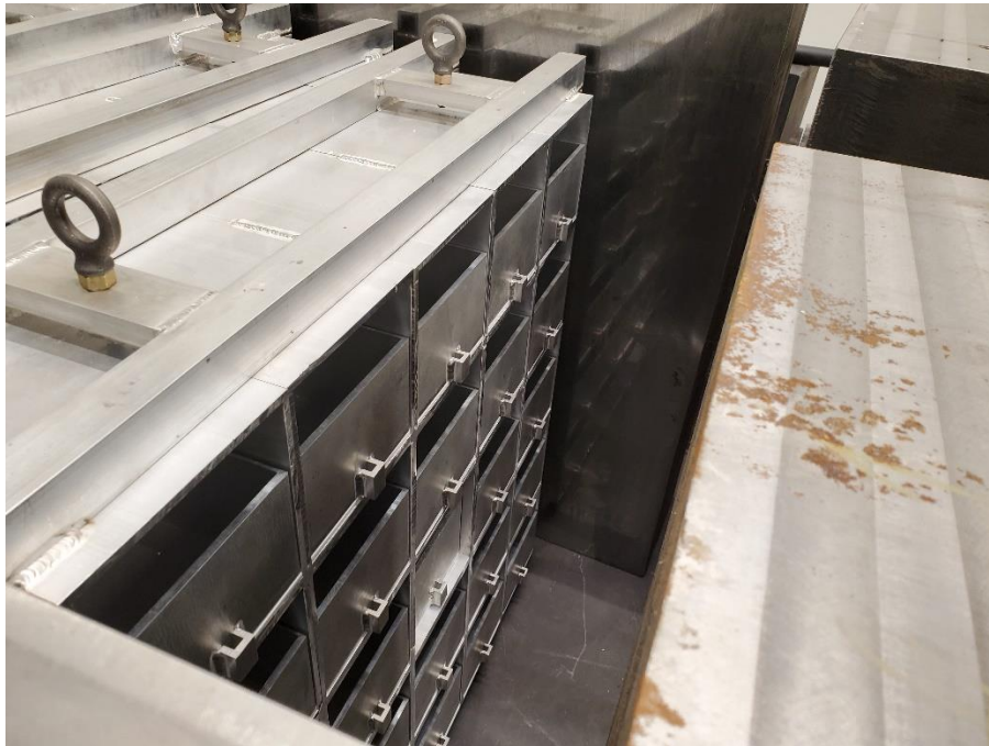
Figure 1.1: FNS Under Construction
