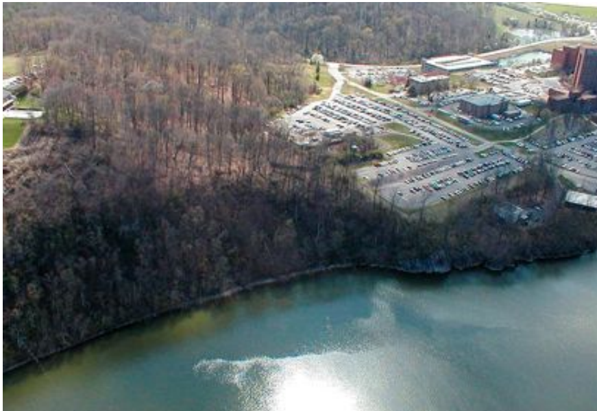
Figure 1. An aerial view of the Anthropology Research Facility. Note the varying elevation of the south waterfront. Photograph taken in March 2001.
