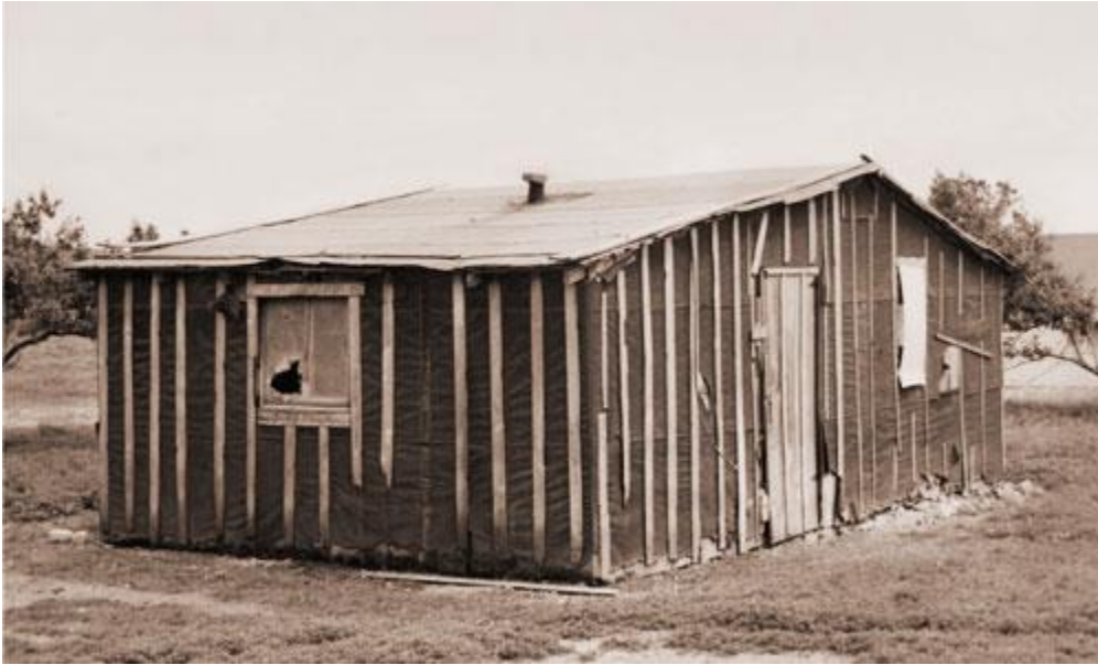
Figure 5.3 Dilapidated Shack (Tyson Foods 2013e)
