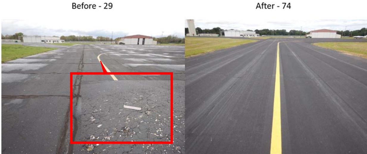
Figure 24. MKL CTJK-004 before and after maintenance repairs
