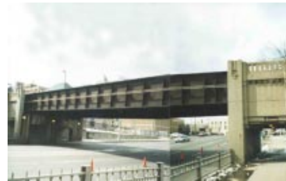
Railroad bridge over Woodward Avenue Source: Author
