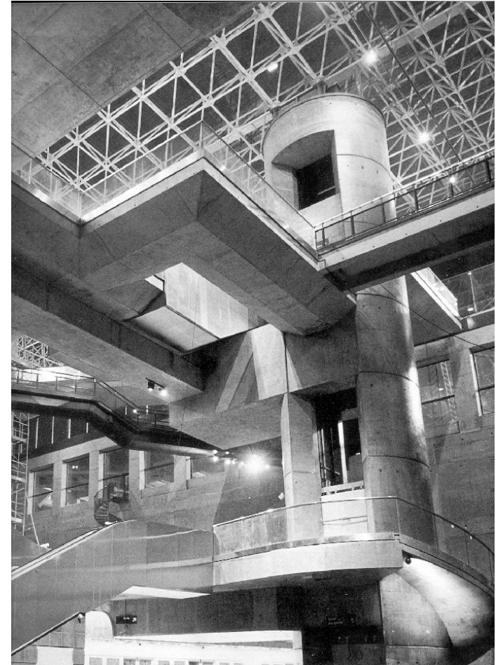
Fig. 39 Photo of elevator tower in Espace-Piranesien Source: Binney, 28
