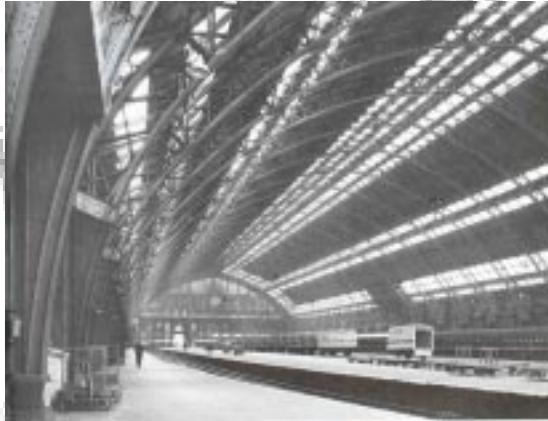
Fig. 49 S. Pancras Station platforms Source: Fletcher, 1125
