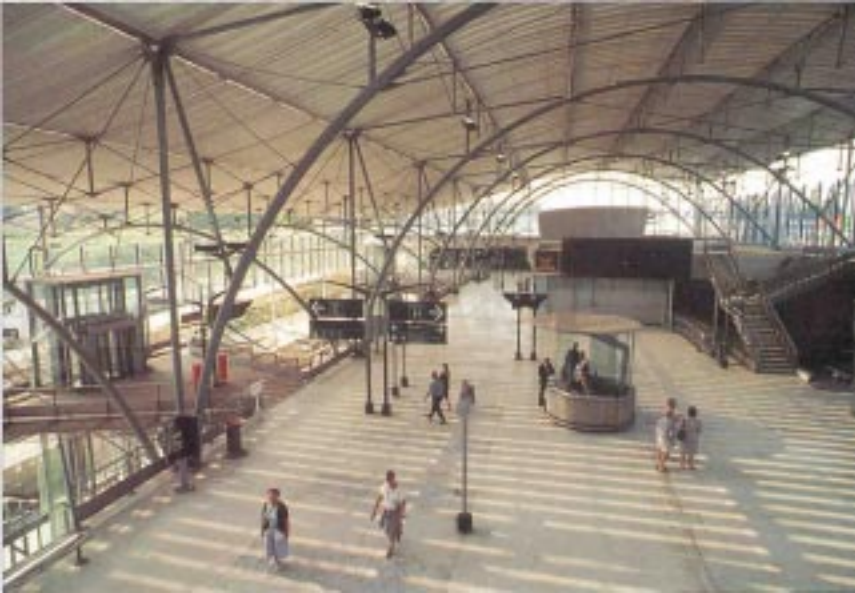
Fig. 38 Photo of Lille-Europe concourse & elevator towers Source: Binney, 30
