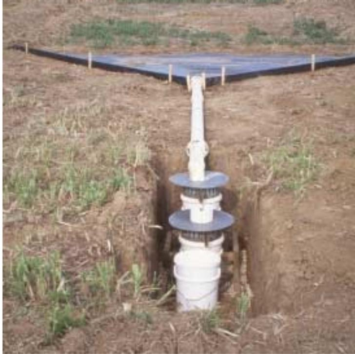
Figure 4. Placement of flow dividing buckets in the sump hole.
