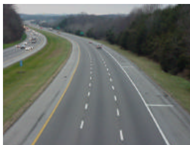
Figure 4-07. McMillan Road overpass (I-40 westbound, looking west)
