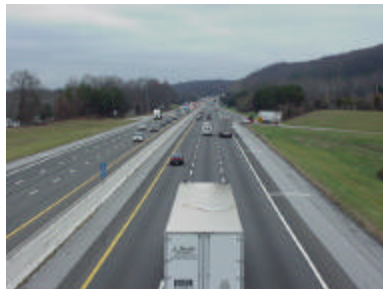
Figure 4-04. Watt Road overpass (I-40 eastbound, looking east)
