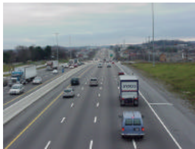
Figure 4-03. Walker Springs Road overpass (I-40 westbound, looking west)
