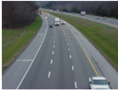
Figure 4-06. McMillan Road overpass (I-40 eastbound, looking west)
