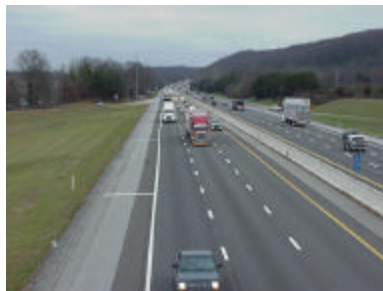
Figure 4-05. Watt Road overpass (I-40 westbound, looking east)
