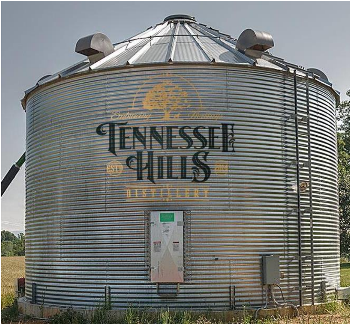
Figure 8. Silo for storing Tennessee Hills Distillery's corn. Tennessee Hills Distillery is bringing a new type of business to a local silo as their demand for corn and corn storage increases in the coming years.
