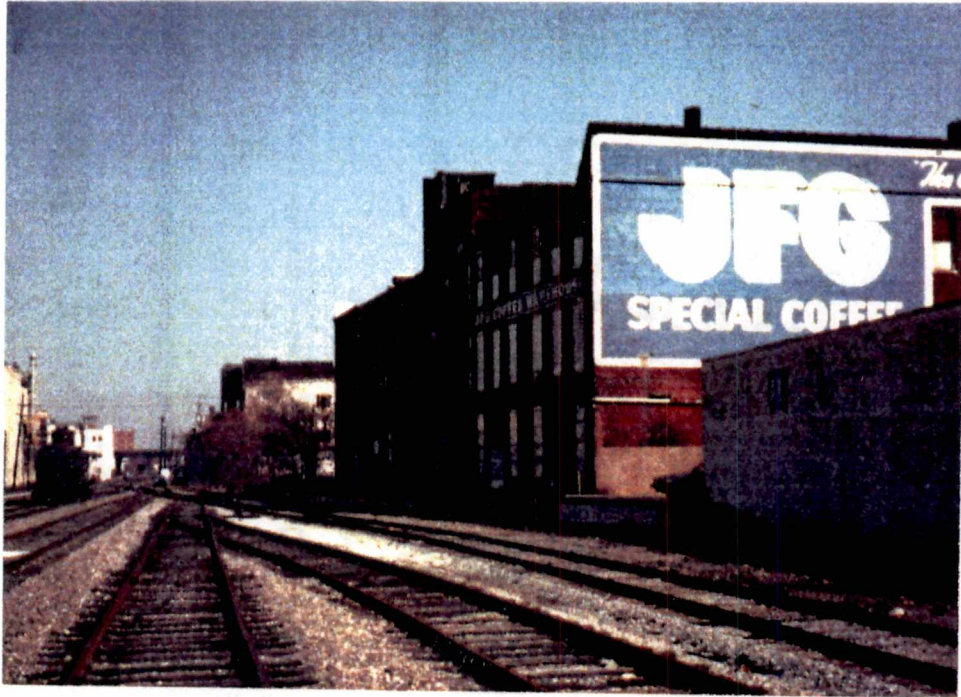
Figure 2.6 - Jackson Avenue Warehouses and Railway Siding Viewed from Northwest
