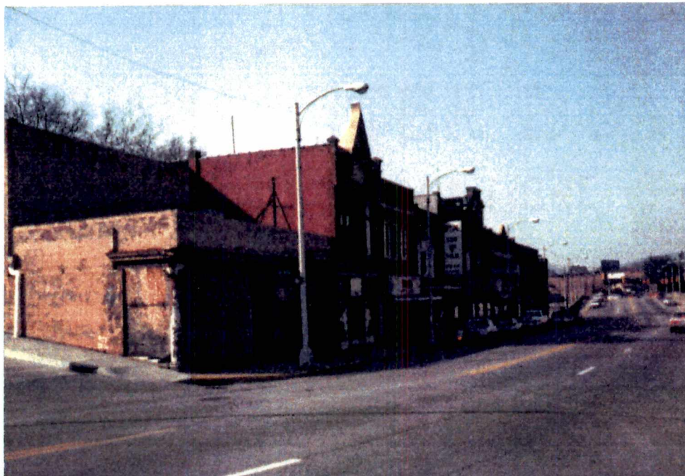
Figure 2.11 - West Side of the 100 Block of Gay Street, 1991 Photo Credit: Craig Nielson
