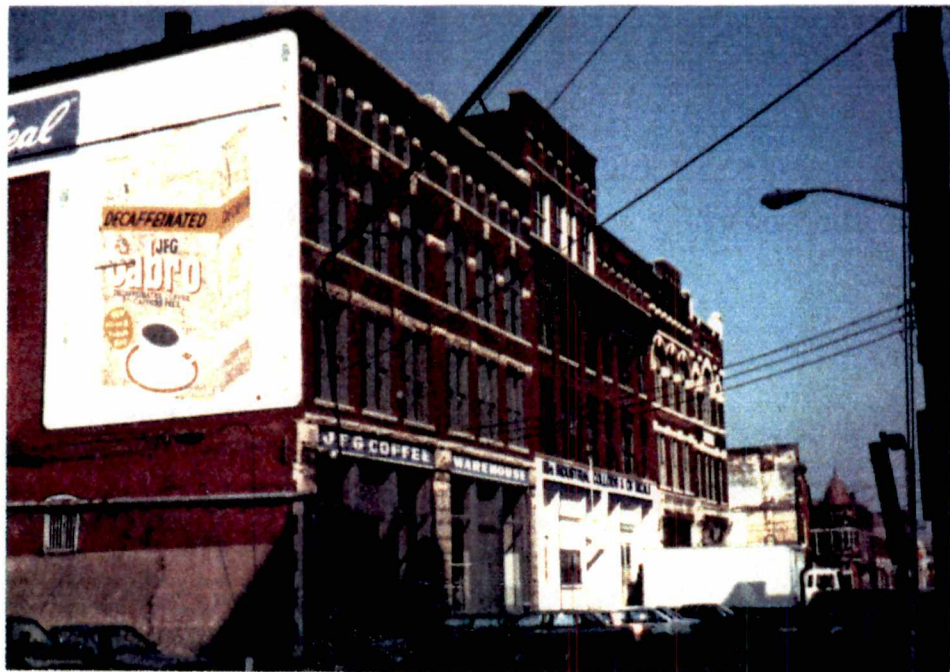
Figure 2.7 - Jackson Avenue Warehouses Viewed from West
