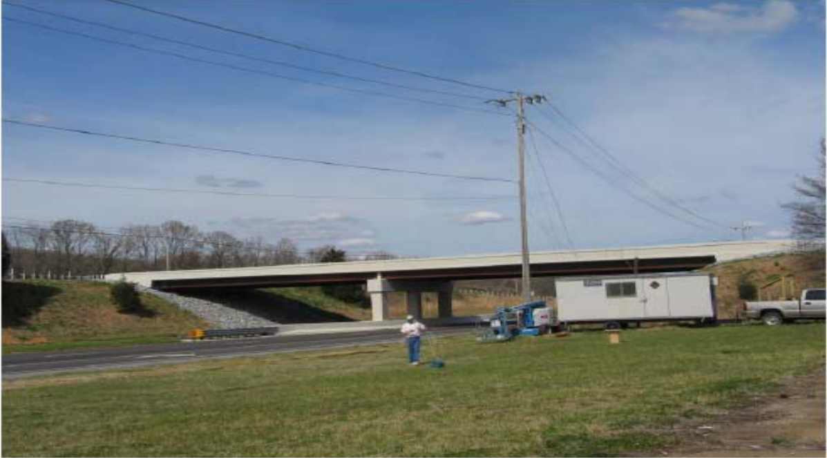
Figure 2.2: Photograph of DuPont Access Bridge Elevation Looking East
