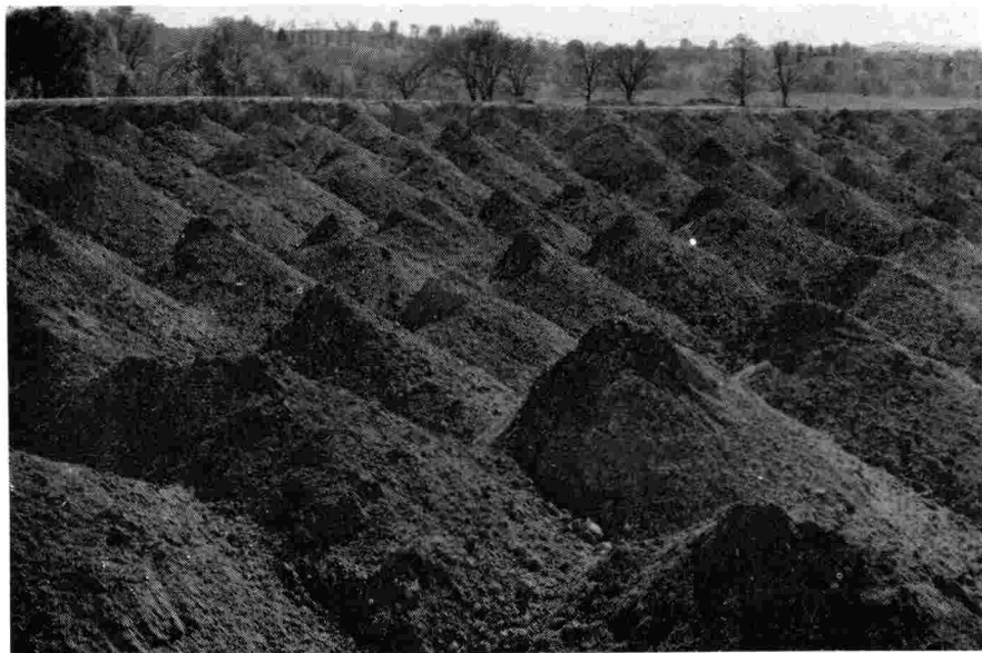
Figure 3. The soil overburden after mining and before land forming operations.
