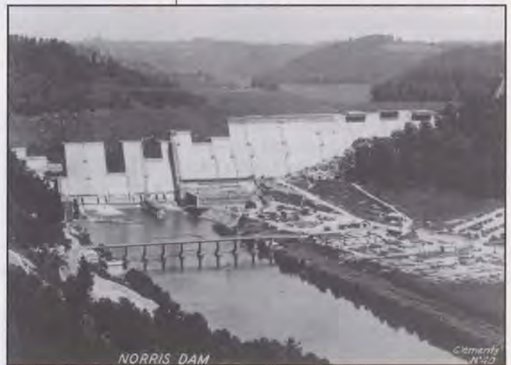
Downstream view of the Norris Dam site in September 1935. Construction of the powerhouse has just started and three overhanging portions indicate the finished height of the dam. Note the cleared valley in the background with the trees representing the future shoreline. (George Palo Collection.)
