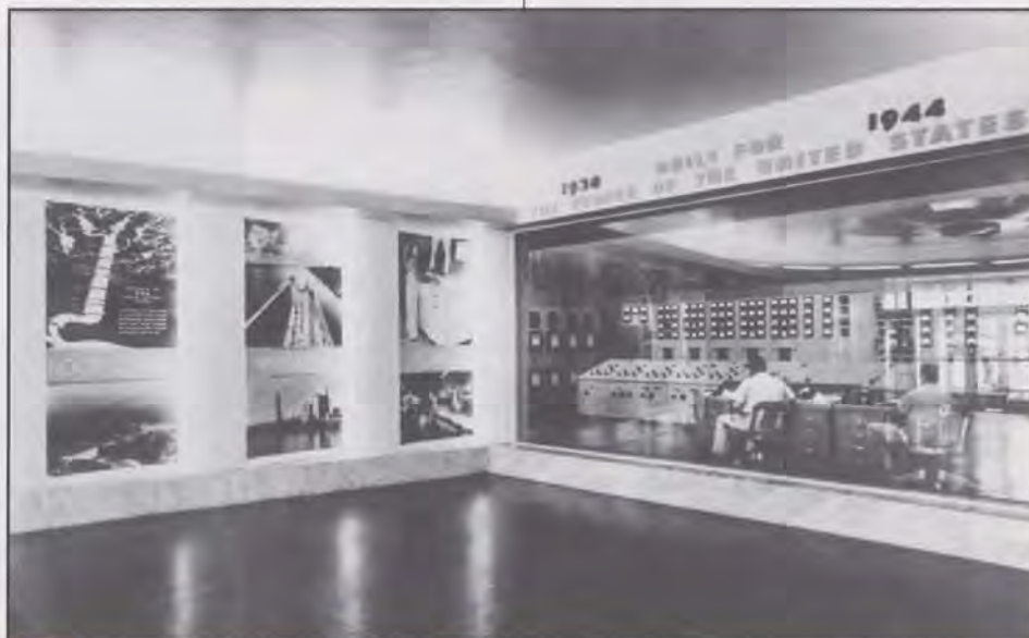
Inside of the Kentucky Dam powerhouse lobby. At a number of dams visitors are able to see workers regulating water levels and power production. On the wall TVA points to Flood Control, Navigation, and Power as its main objectives. (Robert Coe Collection.)
