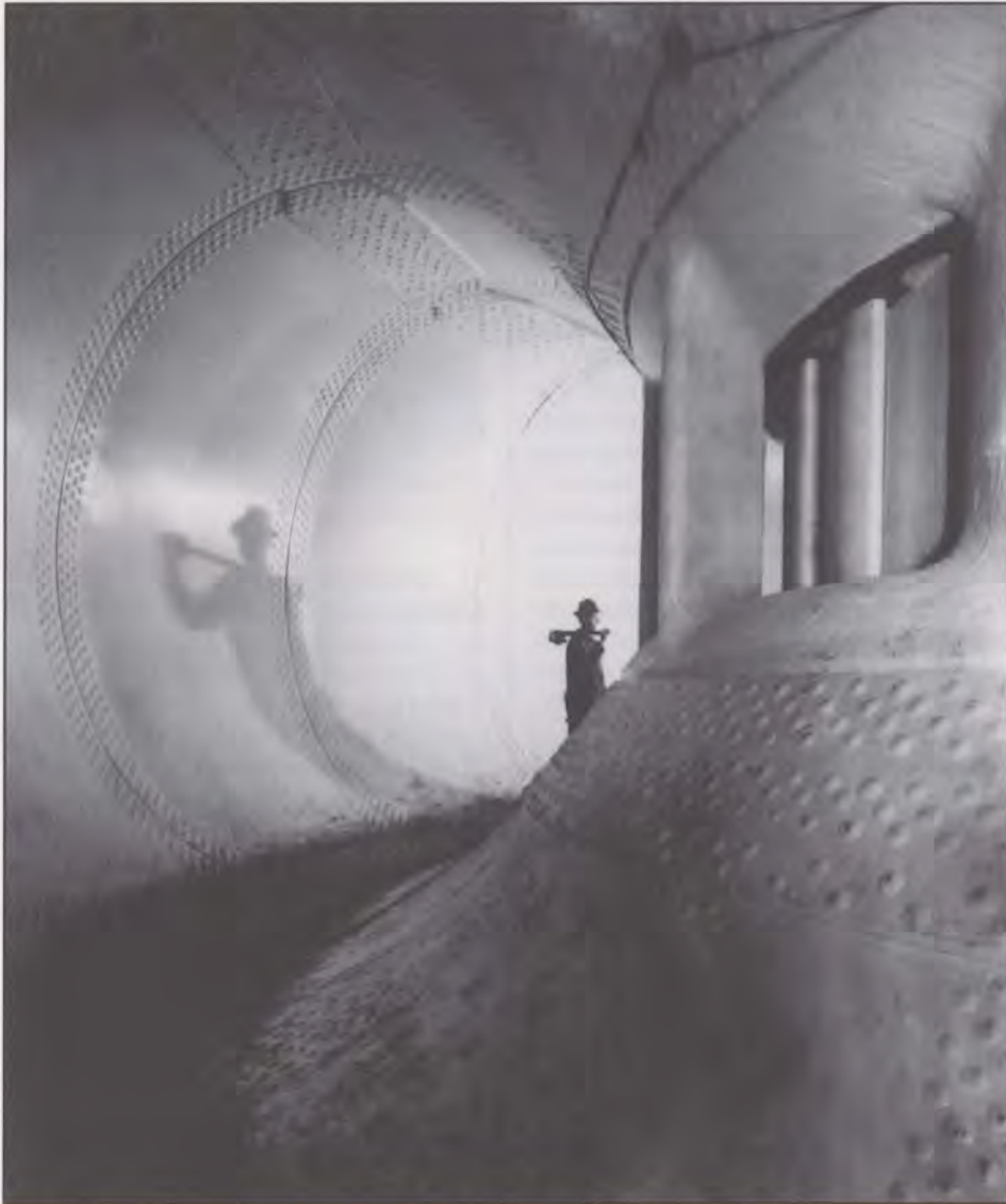
Construction worker inside of Norris Dam turbine, May 1935 (Robert Coe Collection.)
