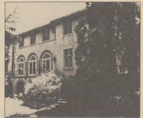
The John Craig house, built in 1926 on Knoxville's Westland Drive is an elaborate and richly appointed example of Charles Barber's work in the Italian villa style, from The Architecture of Barber and McMurry , 1915-1940. (Knoxville: Dulin Gallery of Art, 1976, p. 46.)
