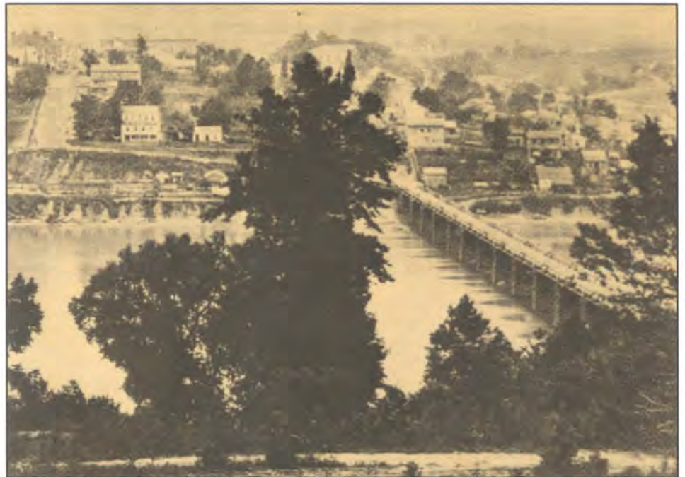
The military bridge at Knoxville built in 1864. (Library of Congress.)
