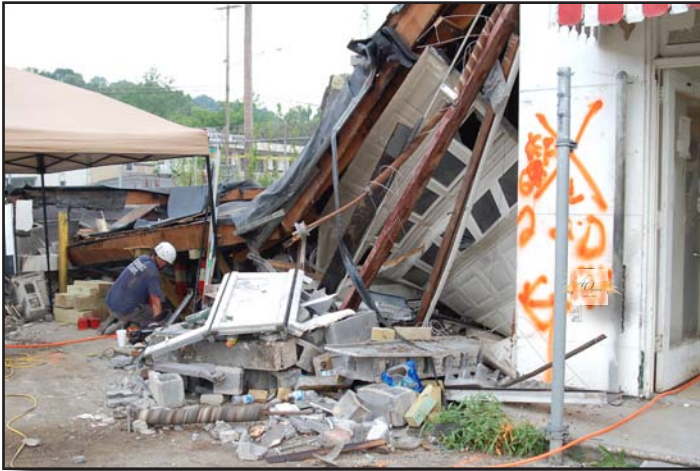
This is a view from outside of the gas station showing the collapsed garage area.
