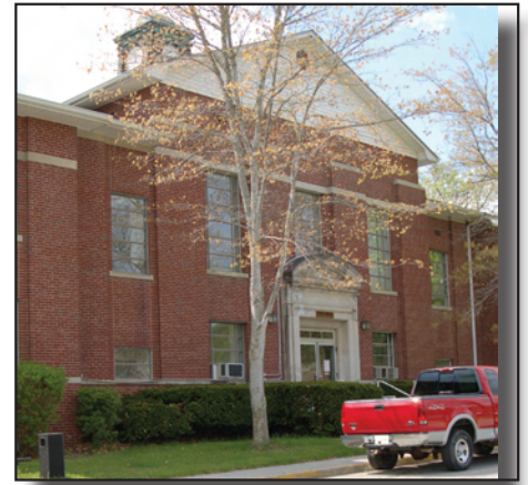
Old Scott County Courthouse
