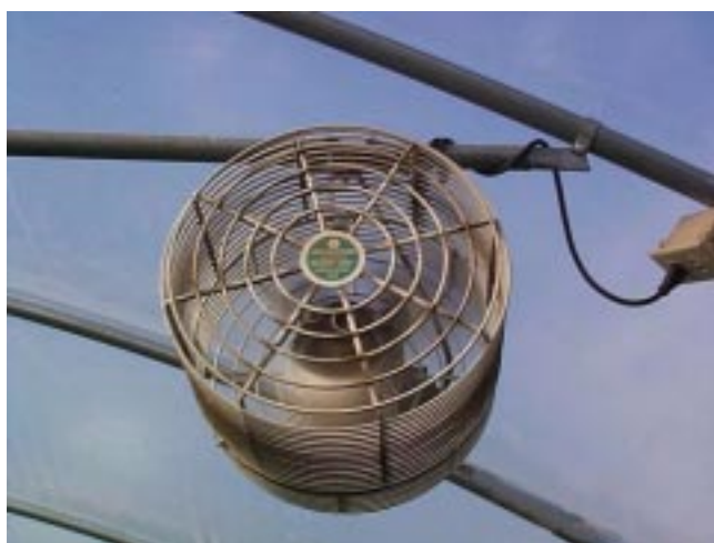
Horizontal airflow fans
