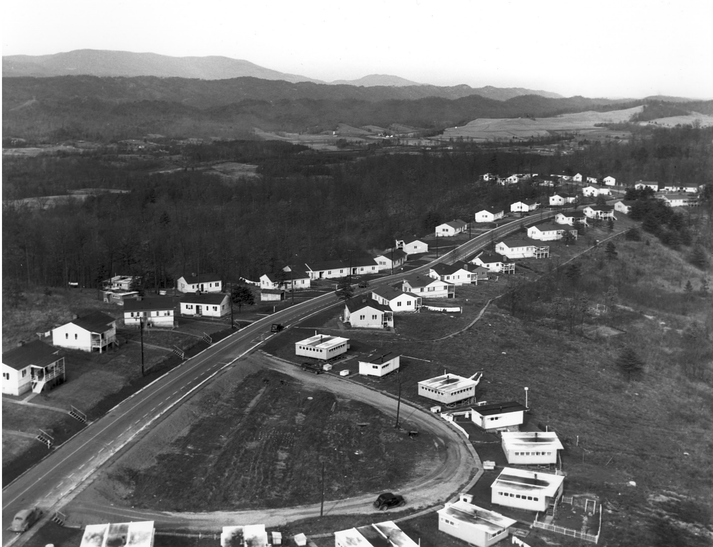
View From Water Tower of Housing in Oak Ridge, 1945
