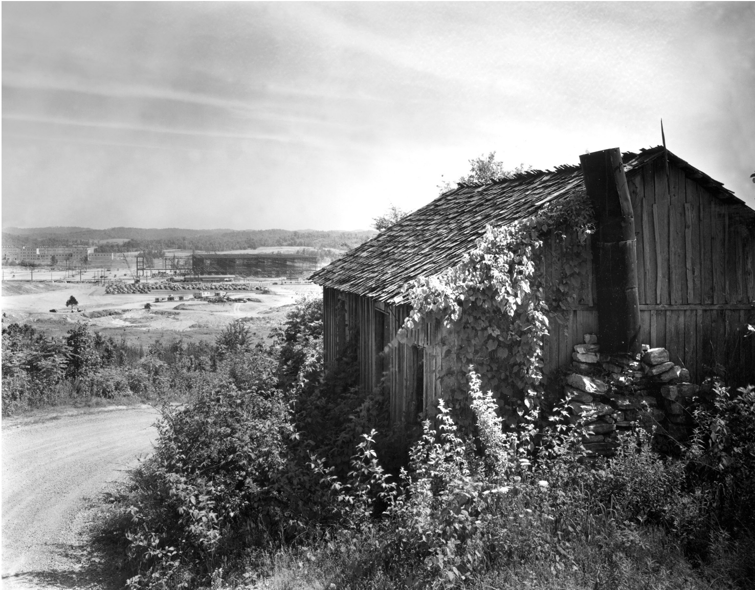
Early Construction of the K-25 Plant with One of the Original Oak Ridge-area Houses in the Foreground, 1942
