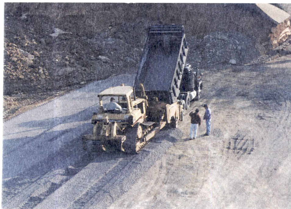
B. DUMPING AND SPREADING THE MATERIALS
