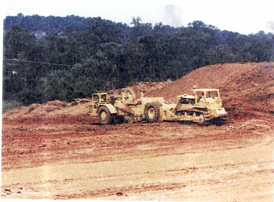
D. SCRAPER WITH A DOZER
