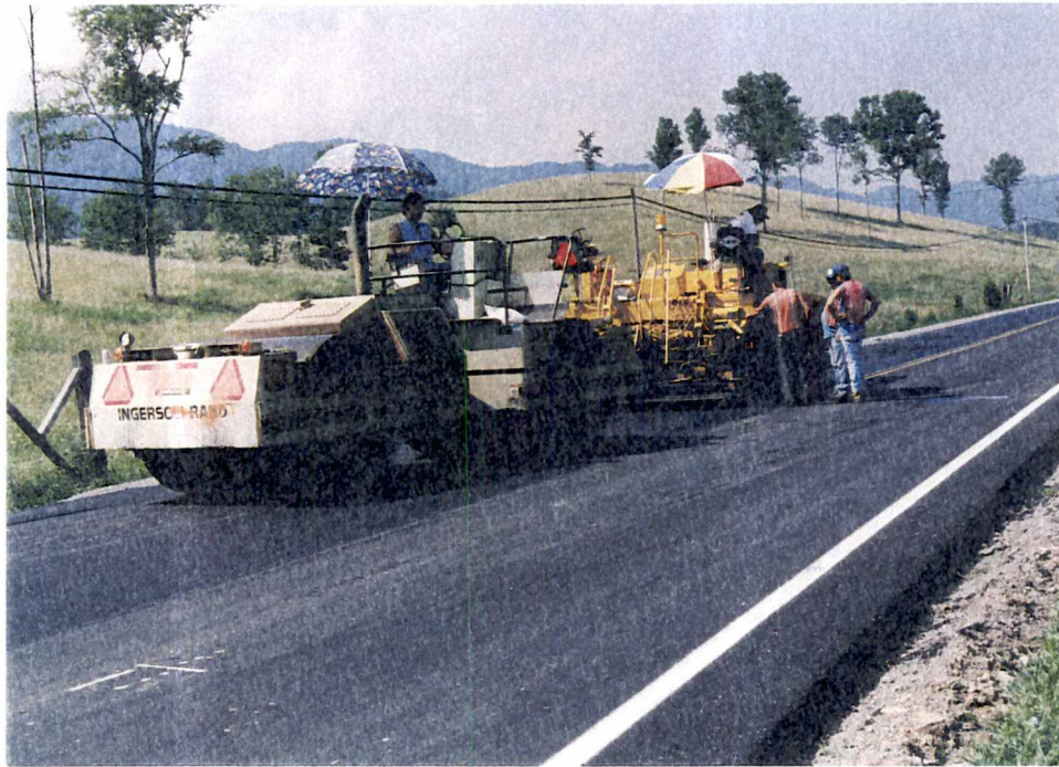
C. COMPACTION (FIRST STEEL ROLLER)
