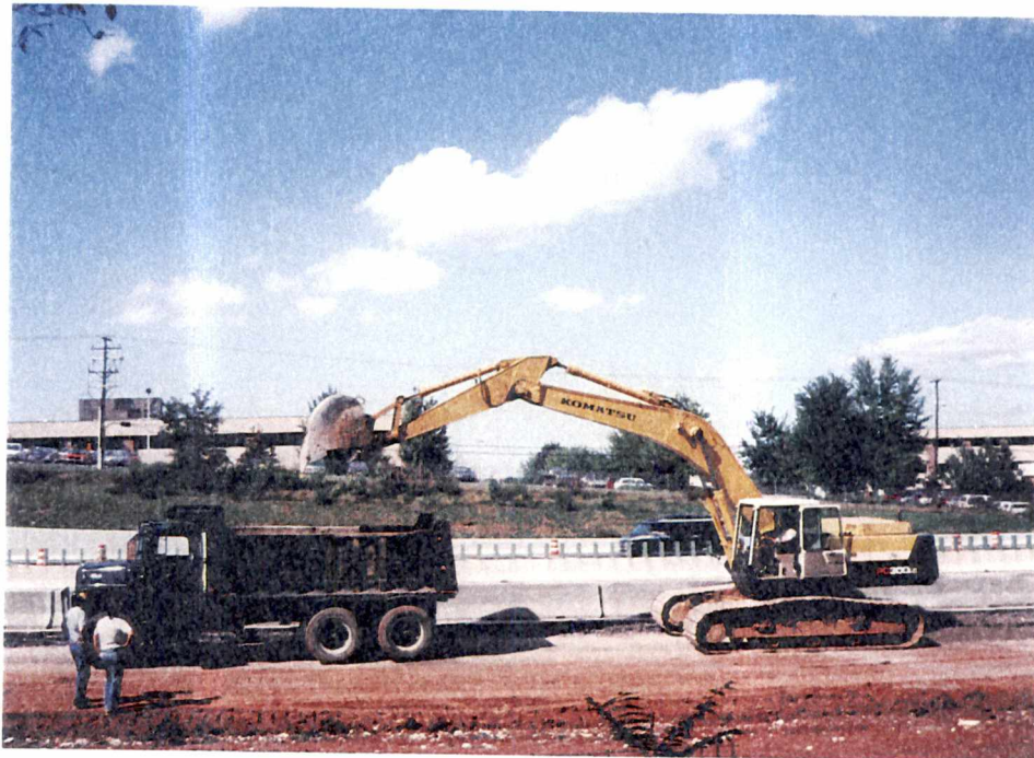
B. TRIAXLE TRUCK AND EXCAVATOR
