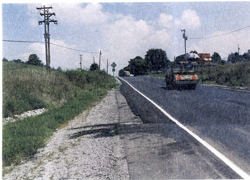
D. COMPACTION (SECOND STEEL ROLLER)
