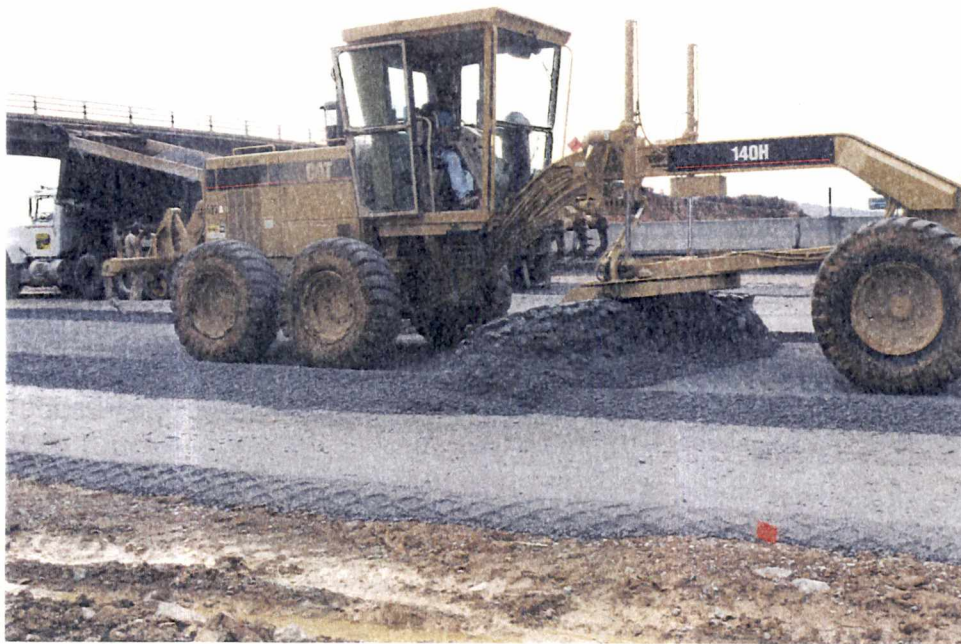
C. GRADING THE MATERIAL WITH A GRADER
