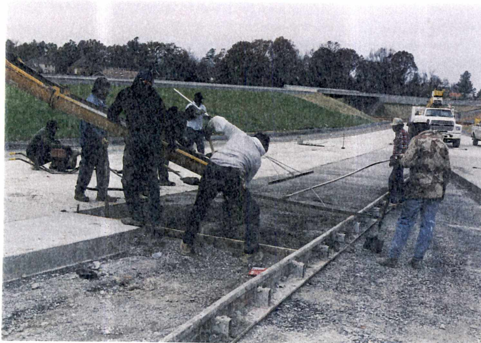
B. FINISHING CONCRETE
