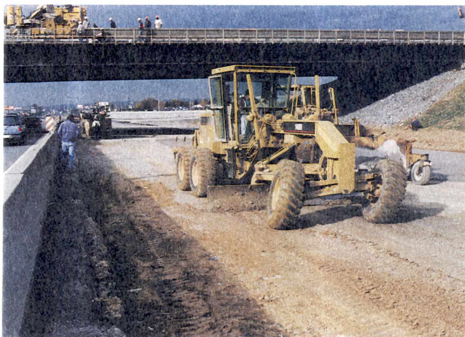
A. SUB-GRADE PREPARATION USING SCRAPER
