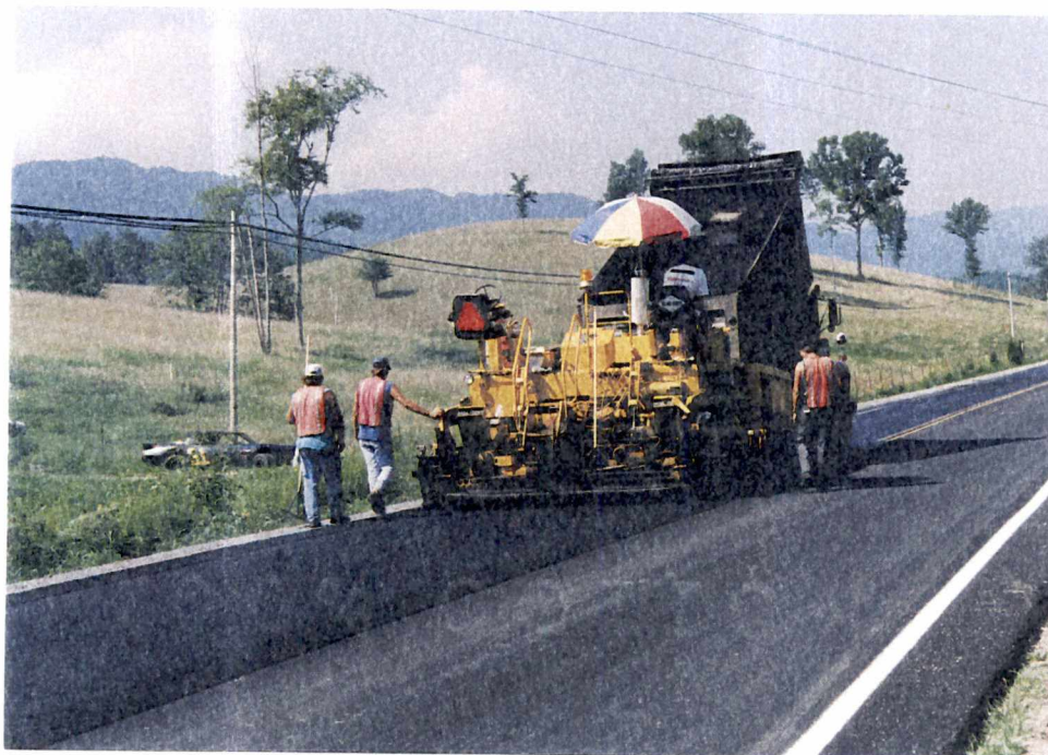
B. DUMPING AND SPREADING THE MATERIAL
