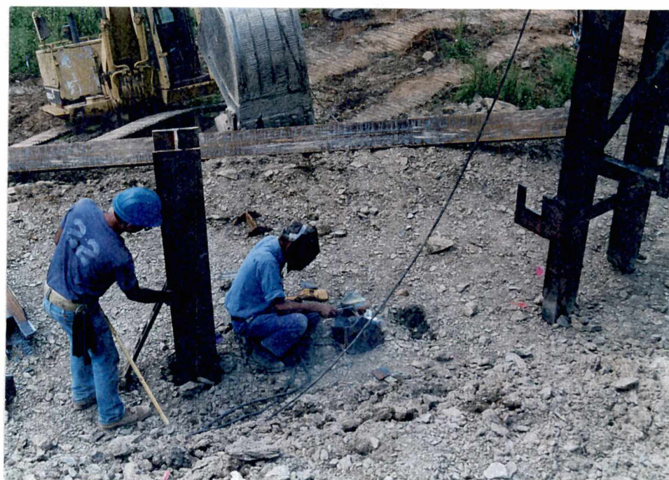
B. WELDING AN EXTENSION TO A PILE
