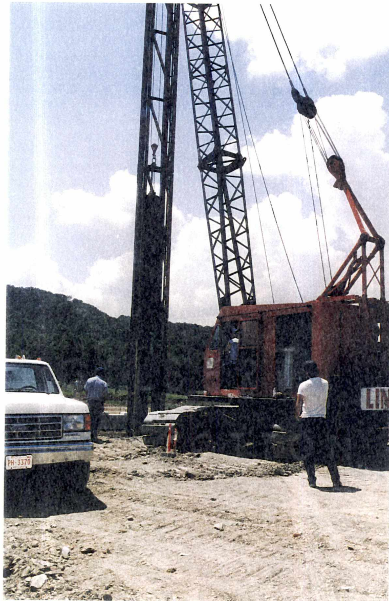
Figure 5-6. Steel Pile Driving
