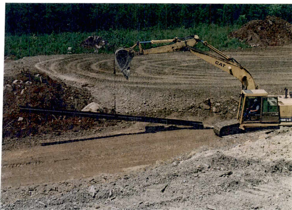
A. EXCAVATOR LIFTING A PILE TO THE CRANE
