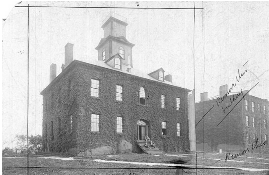
Figure 2. Undated, later photograph of the north façade of Old College, with West College off to the right. Note the presence of ivy, the elliptical fanlight transom over the doorway, and the Serlian window above the transom (the latter two being indications of the Adam or Federal Style). Also note the absence of the cupola. Source: University of Tennessee Special Collections (AR.0018, Box 12, Folder 27), Knoxville, TN.
