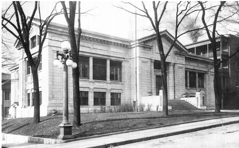
Figure 2. Undated photograph of the Lawson-McGhee Library, Knoxville, TN (completed 1915; demolished), by Miller, Fullenwider, and Dowling, in association with A.B. Baumann. Source: University of Tennessee Special Collections (MS.0951, Box 2, Folder 2), Knoxville, TN.
