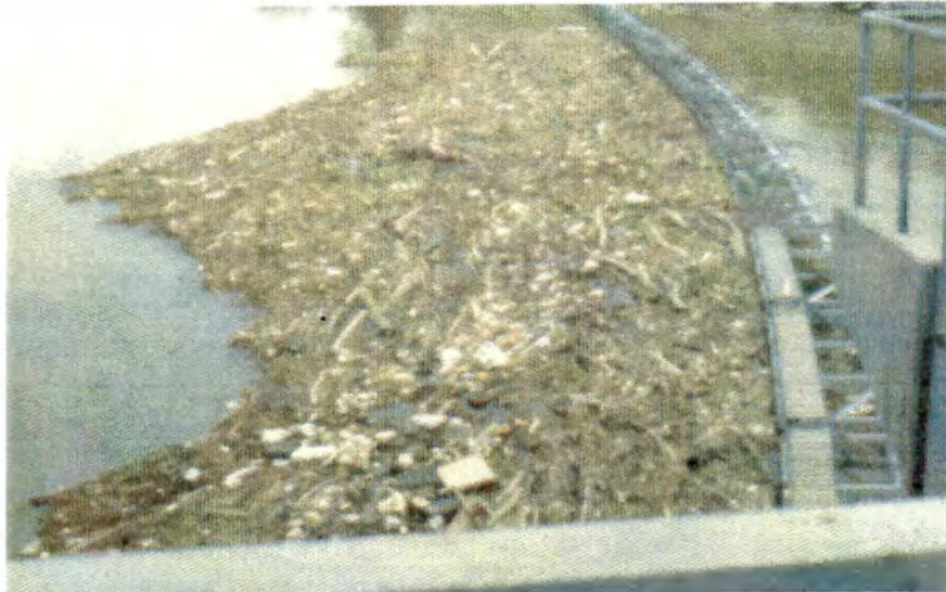
Figure 28. Debris accumulated at Boom at Cheatham Dam
