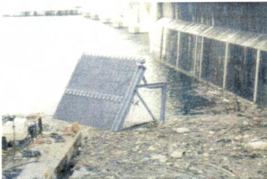
Figure 33. Self-Cleaning Trashracks being installed at Cheatham Dam
