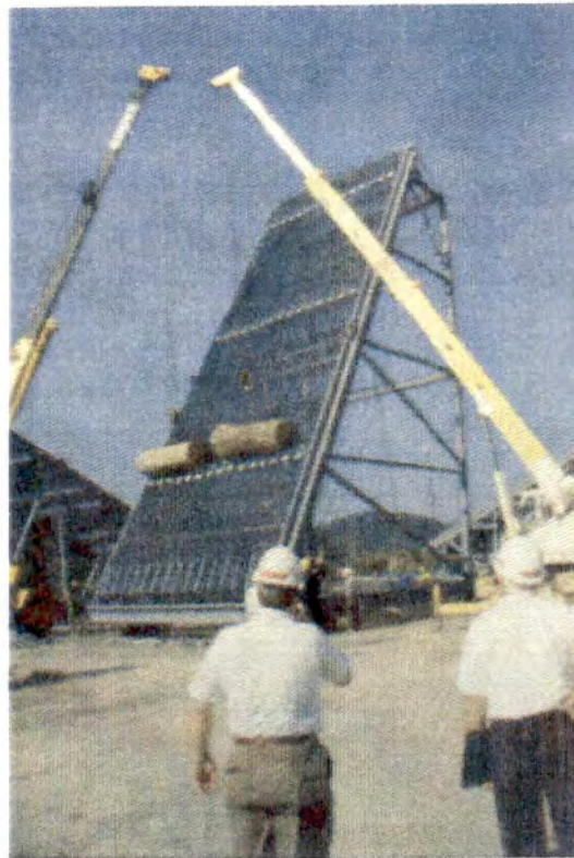
Figure 32. Testing of Self-Cleaning Trashracks
