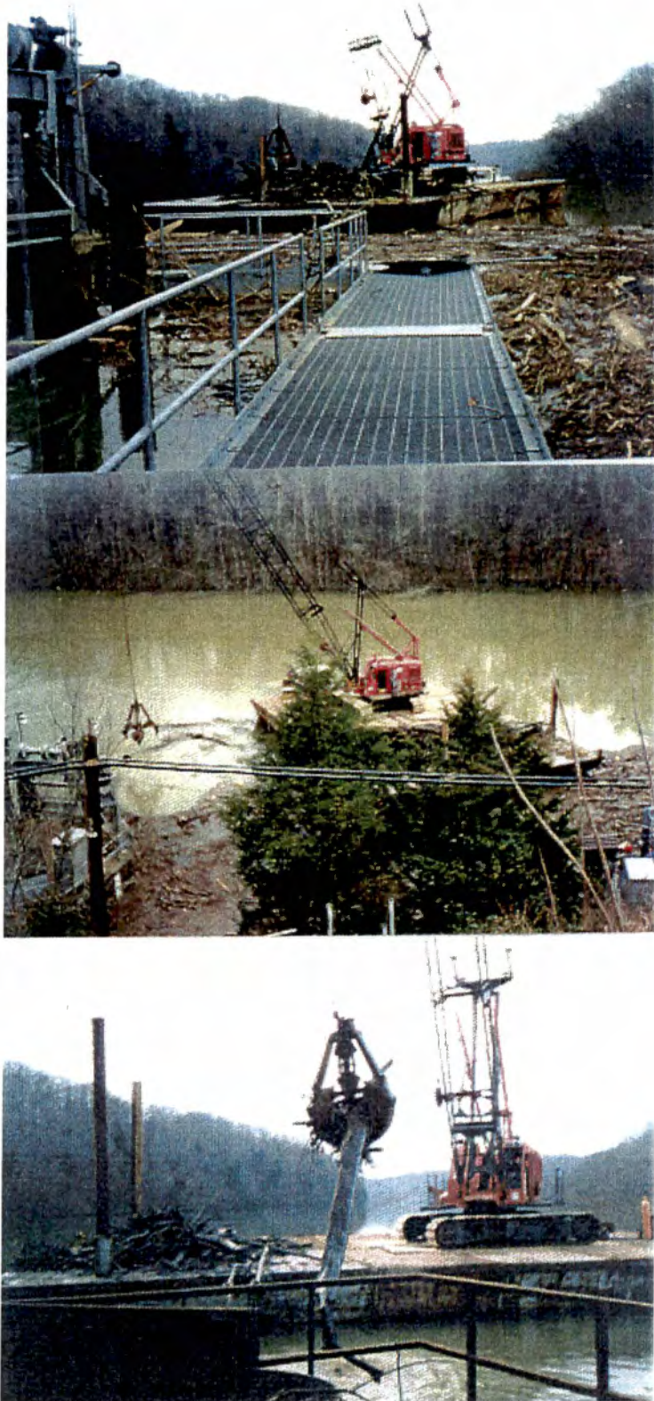
Figure 7. Shows Debris Removal using Barges, Cranes, and Clamshells
