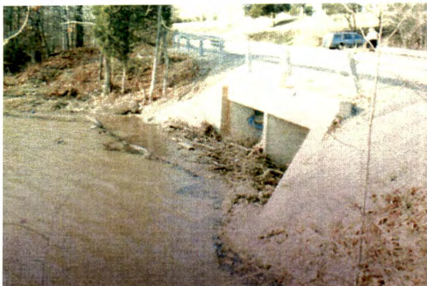
Figure 20. Beaver Debris built in a Spillway Outlet (Ridgetop)
