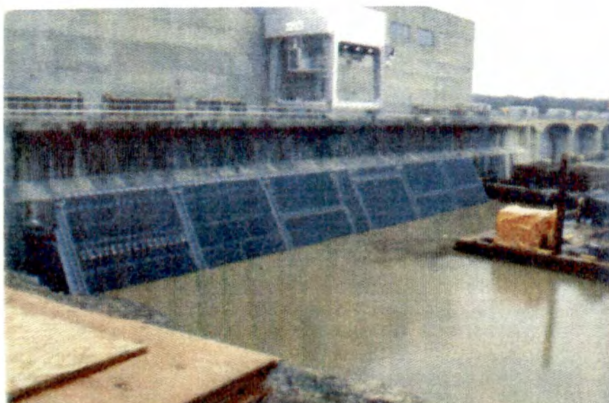
Figure 35. Cheatham Dam Self-Cleaning Trashracks
