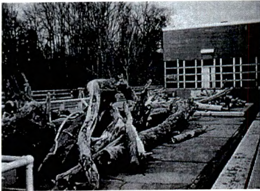
(a) Wheeler Dam – Illustrates the potential size of debris at dam sites (Jones et al., 1997)
