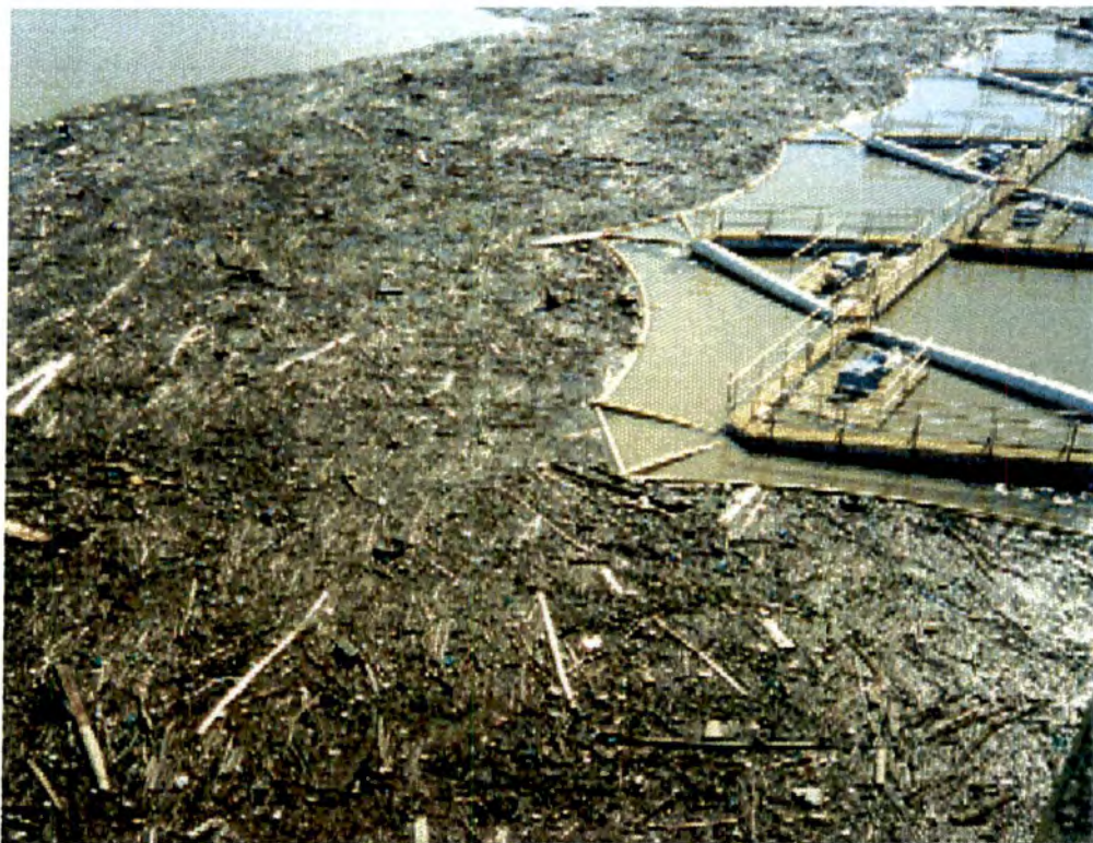
(b) Douglas Dam – Shows booms around aeration pumps (Jacks, 1999)
