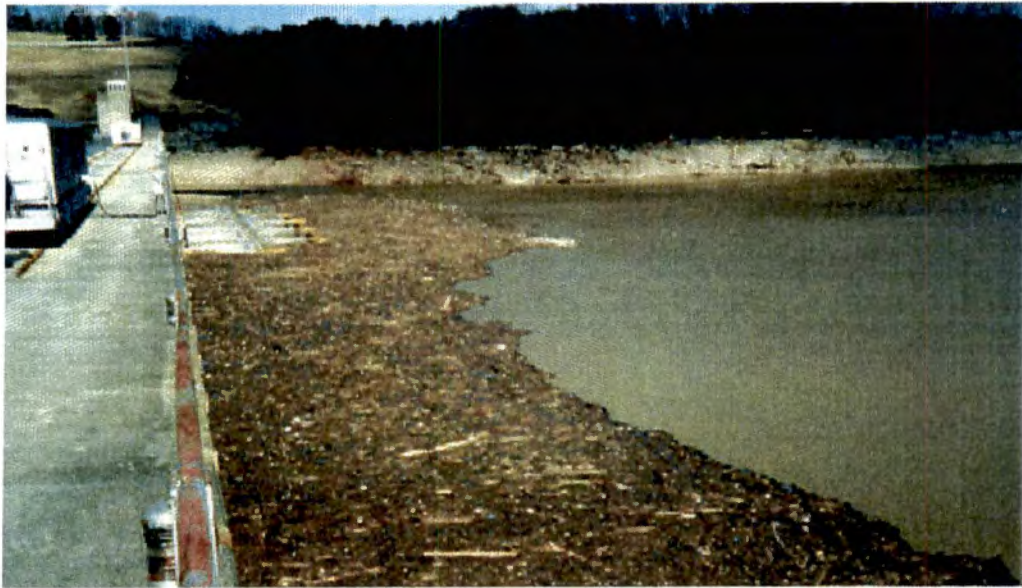
(a) Douglas Dam – Shows debris accumulation and location of aeration pumps (Jacks, 1999)
