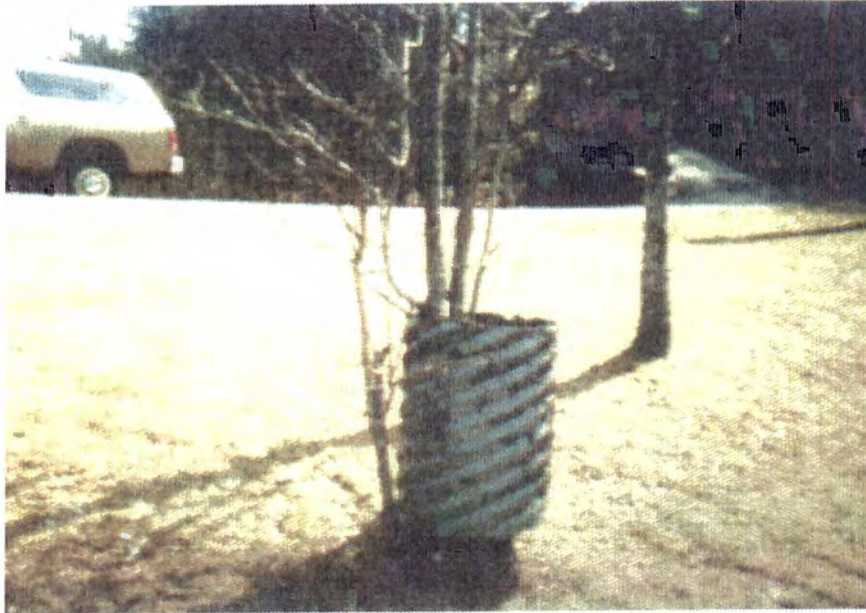
Figure 18. Tree Growing in a Riser Pipe
