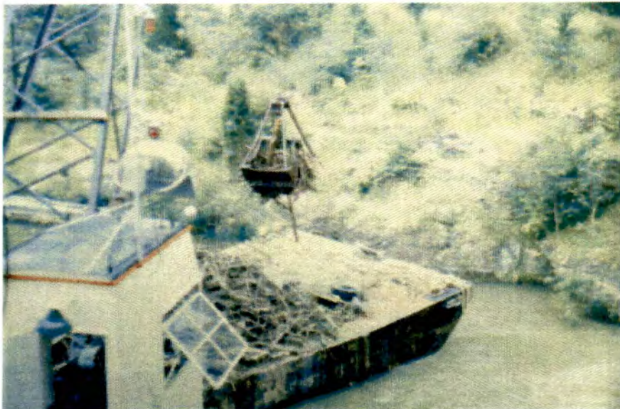
Figure 29. Debris being removed at Cheatham with Crane and Barge
