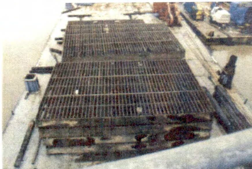
Figure 31. Trashracks Removed from Cheatham Dam
