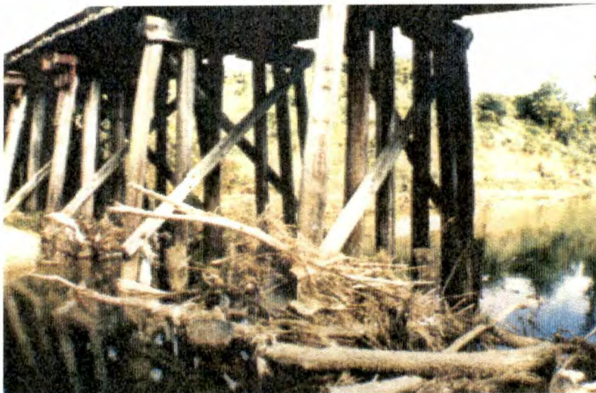
Figure 39. Debris at Piers on Huntsville Springs Branch
