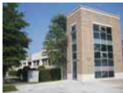
fig. I.23 concrete and brick
