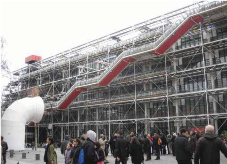
fig. 1.25 view of plaza and exterior escalator tube
