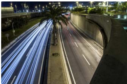
Figure 29 – Bridge Connections. Ronda Litoral, Barcelona.
