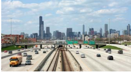
Figure 69 – Dan Ryan Expressway. 12 lanes, 2 service roads, and 2 rail lines.
