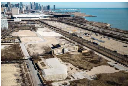
Figure 66 – Remnant(s) of Michael Reese Hospital. Note the rail lines, marshalling yard, and Lake Shore Drive acting as a barrier to the waterfront.
