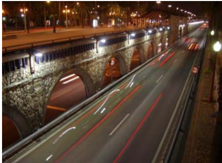
Figure 28 – Multi-Layered Roadways. Public space over highway. Ronda Litoral, Barcelona.
