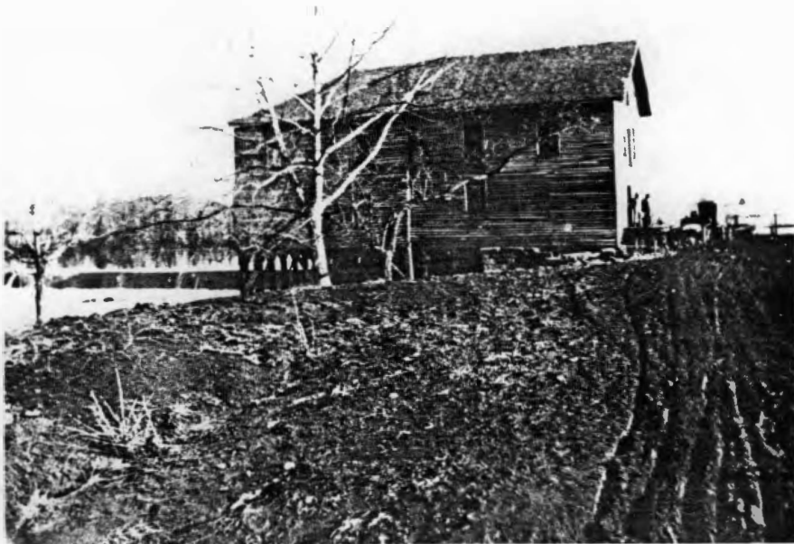
Figure 25. Bird's Mill. Mill is Expanded and the Turbine Bay is Fully Covered. Photograph is Undated.
