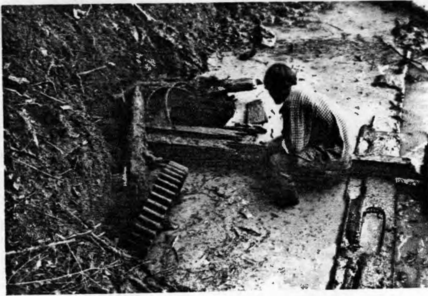
Figure 17. Recovery of Brainerd Turbine. Wooden Sill at Right Extends to Dam. Large Spur Gear in situ.
