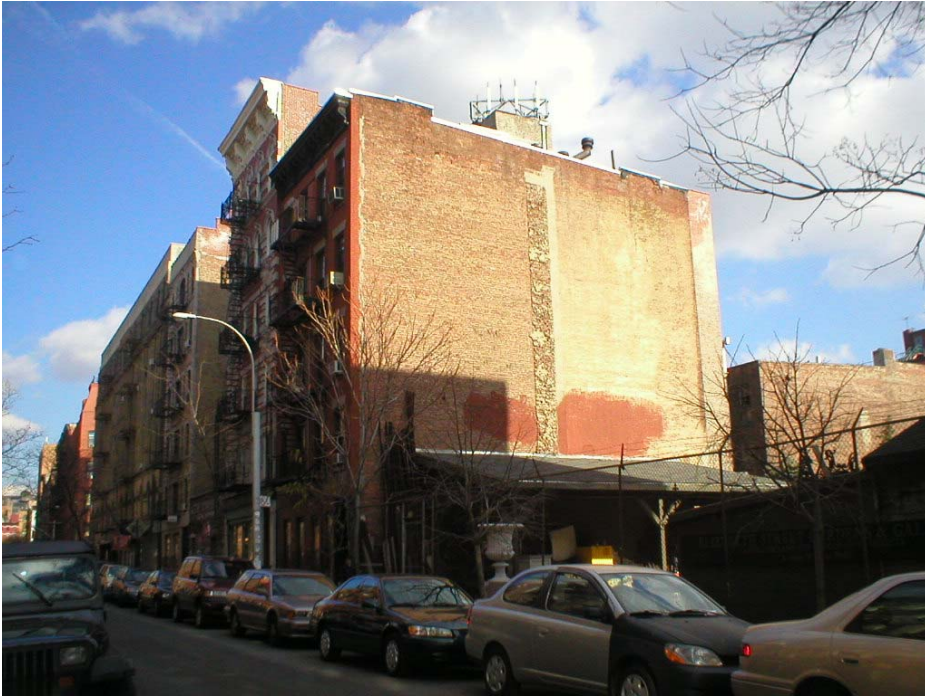
Figure 13. Adjacent Site Buildings - Mott Street (Author)
