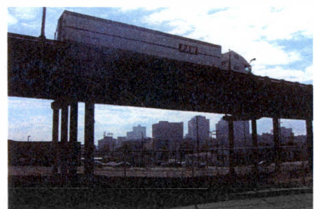
Fig. 2.4 Site photo. Infrastructure 2 Source: Author
