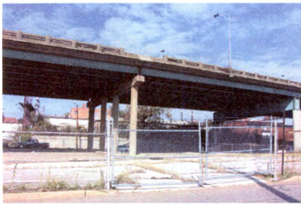
Fig. 2.1 Site photo . Field condition Source: Author
