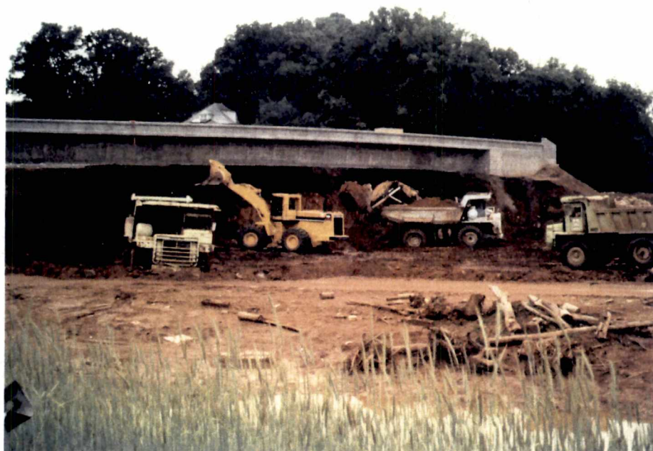
Figure 4.9 Removal operation continued
