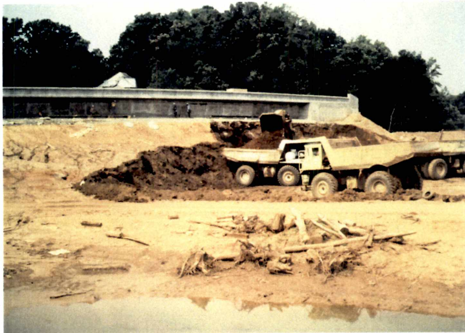
Figure 4.8 Starting removal operations
