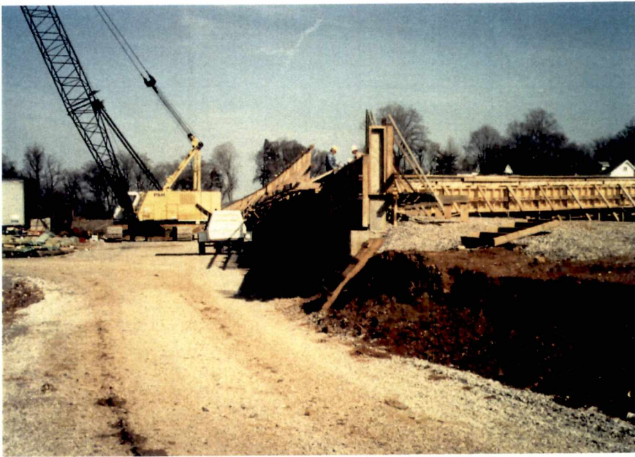
Figure 5.3 Earth shoring height
