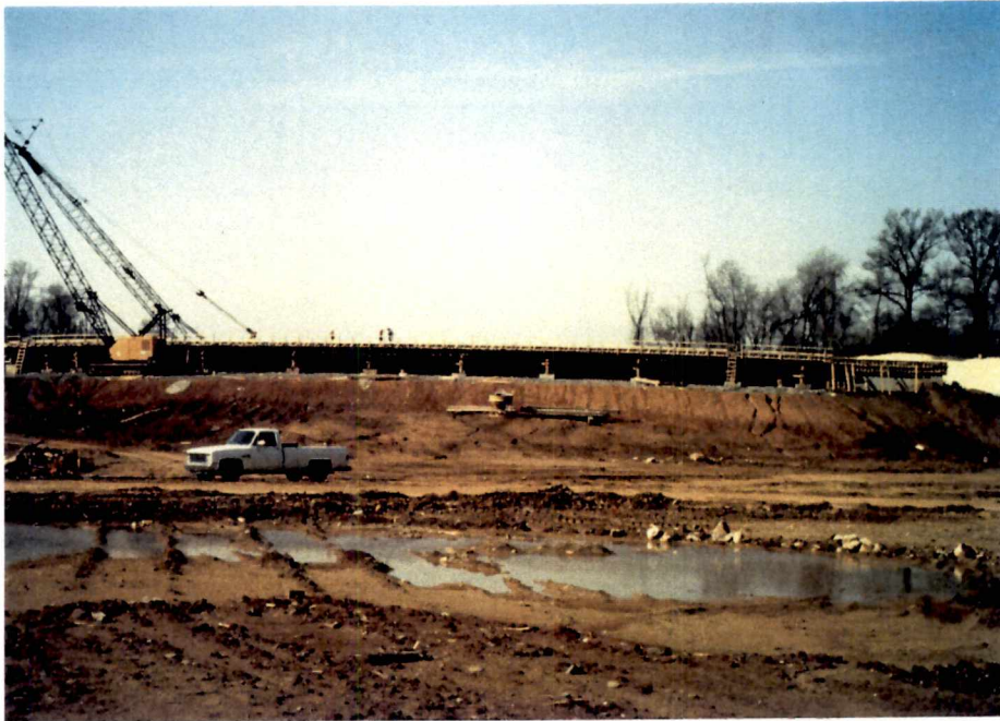
Figure 1.3 Earth shoring embankment
