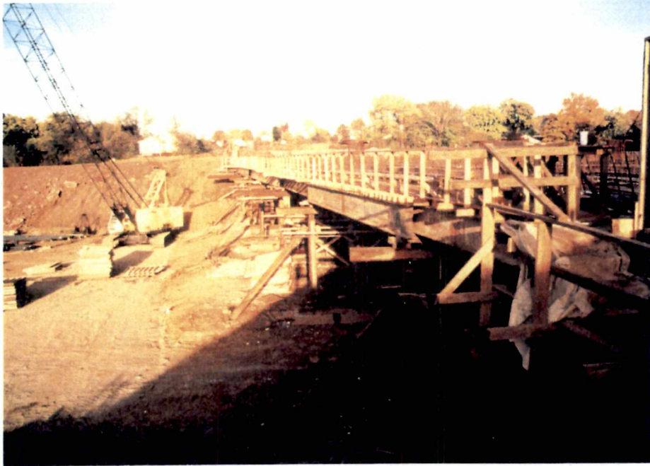
Figure 5.2 Conventional falsework height
