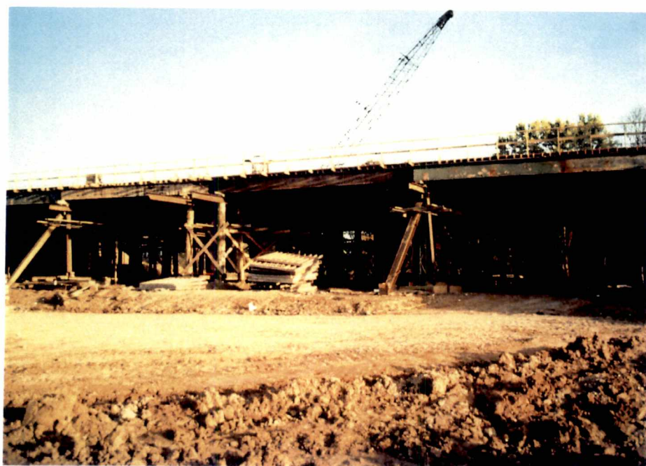
Figure 1.1 Conventional falsework
