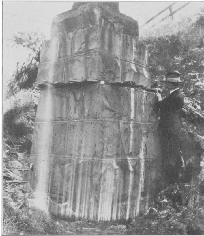
Figure 2.6 Cracking Damage of a URM Pier of Dos Pueblos Viaduct after 1925 Santa Barbara Earthquake (Kirkbride 1927)
