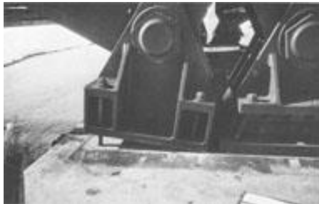
Figure 2.10 Anchorage Failure at the Bearing of a URC Pier of Bridge 14.5 after 1964 Alaska Earthquake (McCulloch and Bonilla 1970)
