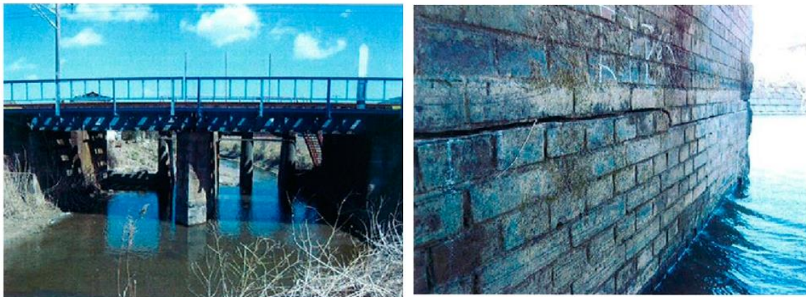
Figure 2.2 Damaged Railroad Bridge and the Crack at the Pier (Abé and Shimamura 2014)
