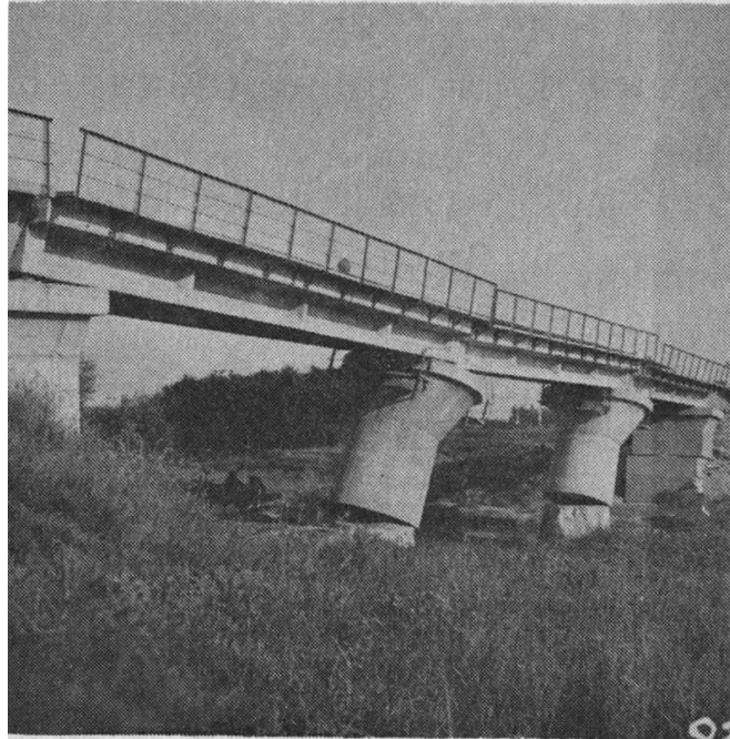
Figure 2.8 Tilting of Upper Partition of URC Piers of Dou River Railway Bridge after 1976 Tangshan Earthquake (Chen 1978)
