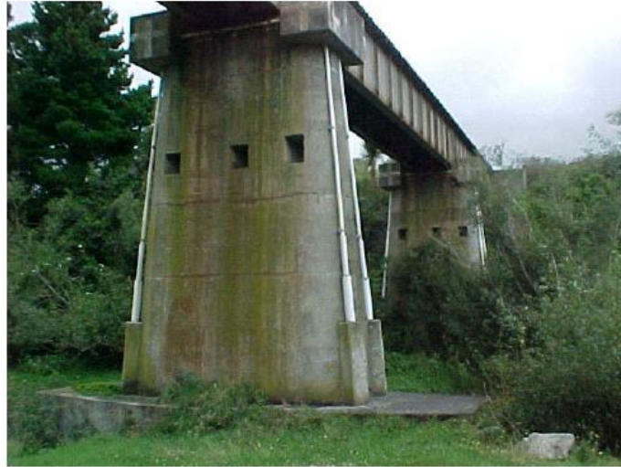
Figure 2.14 External Prestressing Retrofit at a URC Railroad Bridge Pier in New Zealand (Walsh 2002)
