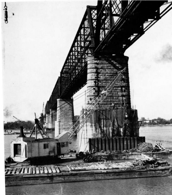
Figure 2.13 Construction of the RC Jacket Retrofitting at a URM Pier of the Illinois Central Railroad Cairo Bridge over the Ohio River (Modjeski and Masters 1953)
