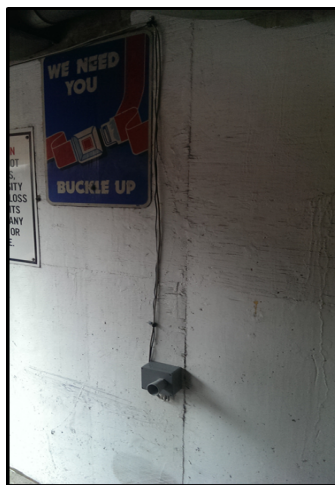
Figure 9. Box housing Sensor #2. RS-232 extension cable and power cable are being fed in from above.
