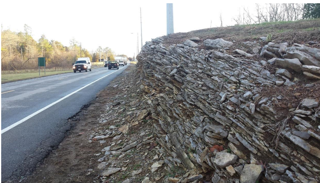
Figure 3: A road cut near Oak Ridge National Lab and Y-12 National Security Complex, showing the 45° dip of the shales.
