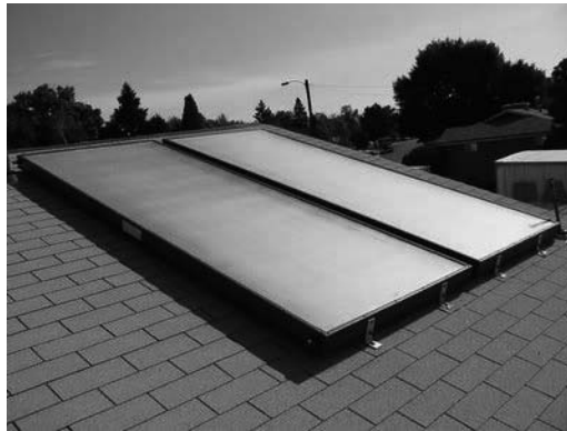
Figure 6-3. A Typical Roof-Top Solar Collector (courtesy of U.S. Dept. of Energy)
