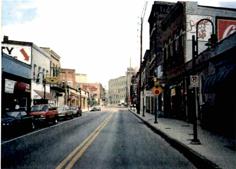
Figure 17 - Central Street looking north approximately 300 feet from the STOP
