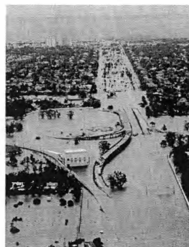
FIGURE 2: AERIAL OF NEW ORLEANS FLOOD
