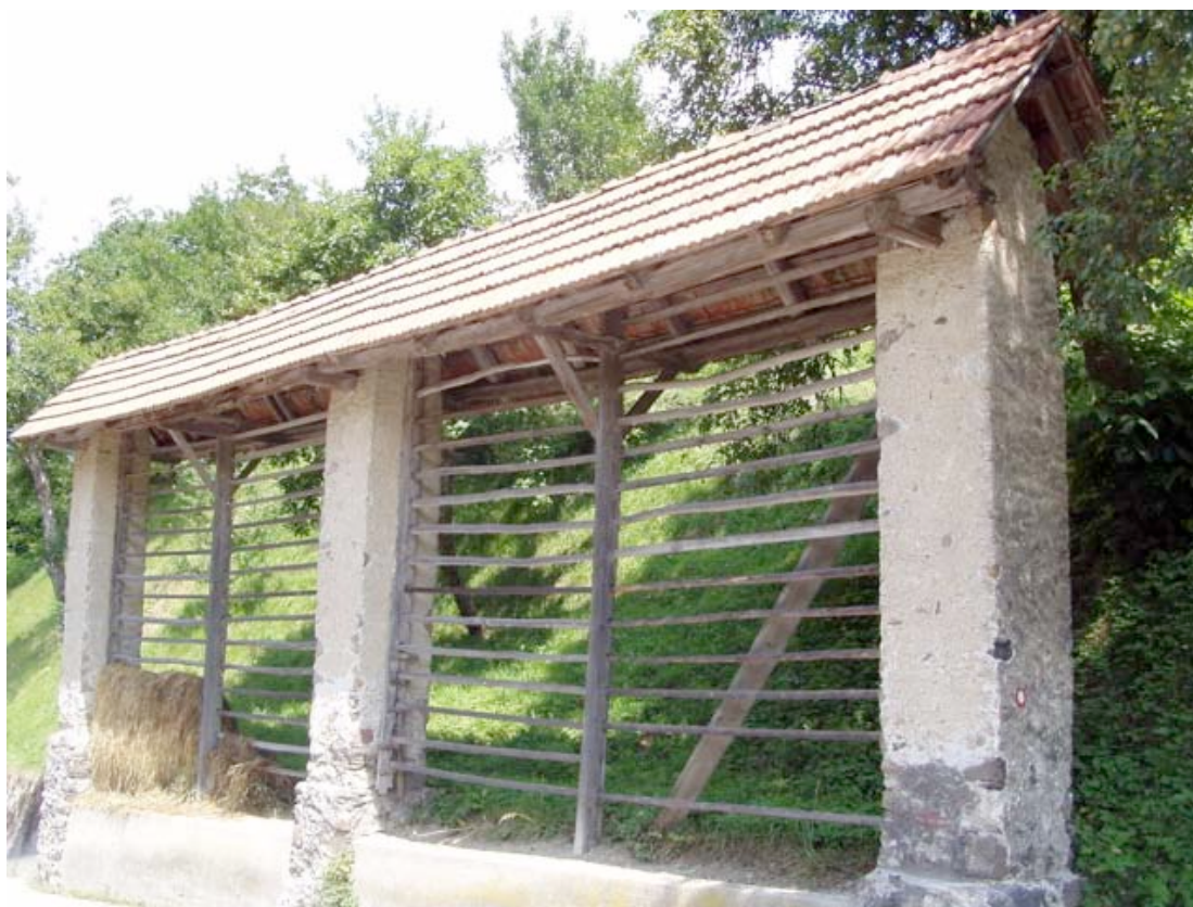
Figure 3. Enojni stegnjeni kozolec z zidanimi stebri. Cerkno, Slovenia. Photograph by Author.
