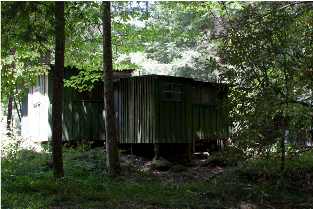
Cabin in disrepair Image by J. Wessels, 2012
