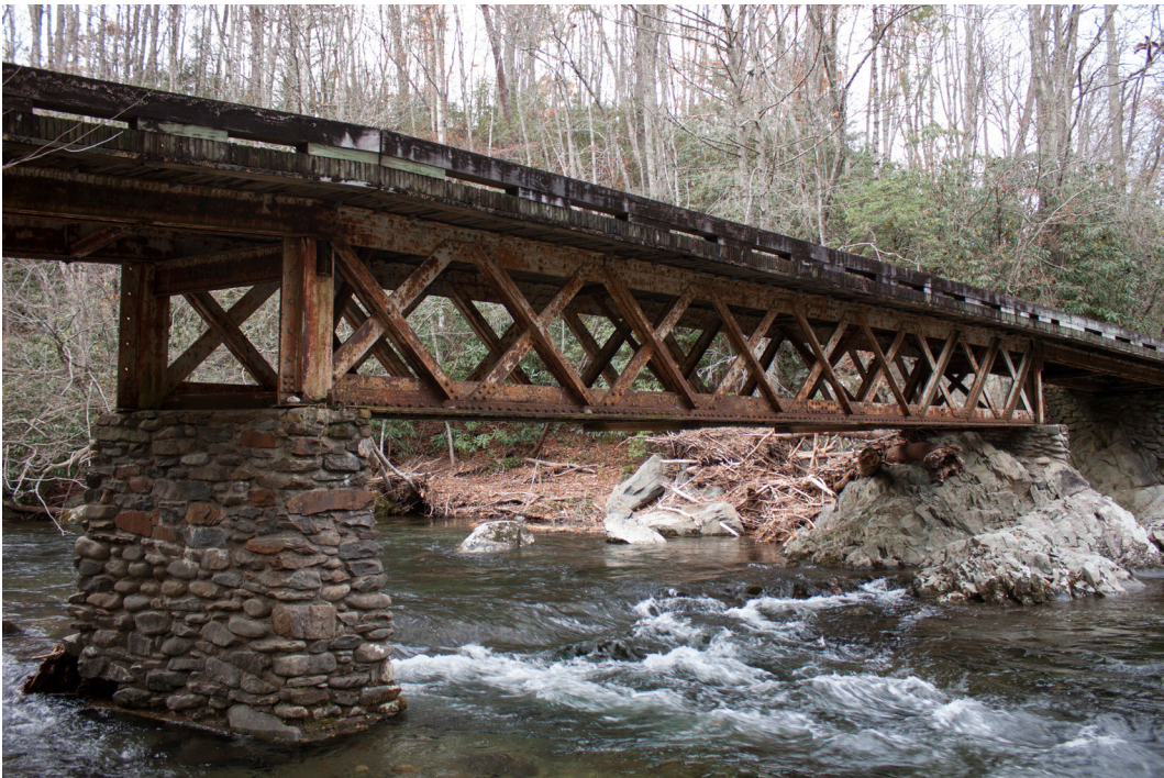
Bridge spanning Little River Image by J. Wessels, 2014
