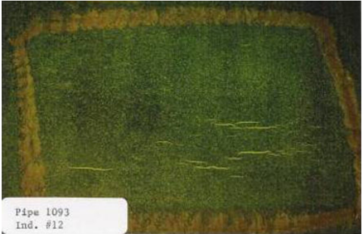
Figure 1.2: Fluorescent MPI image of an SCC colony from a decommissioned natural gas pipeline. The box around the SCC colony is 6\frac{1}{4} inches long by 4 inches wide.
