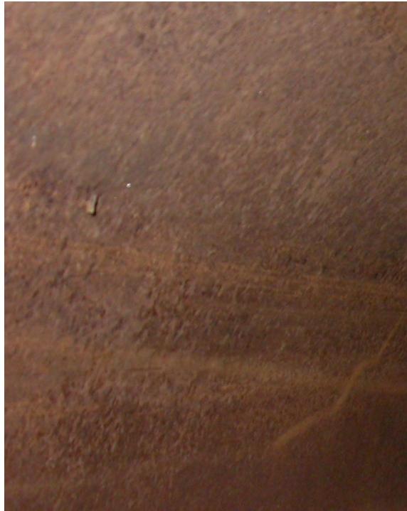
Figure 2.6: This was taken from inside a 30-inch diameter test pipe containing real SCCs. The image is of an approximately two feet wide three feet tall area of inside pipe wall.
