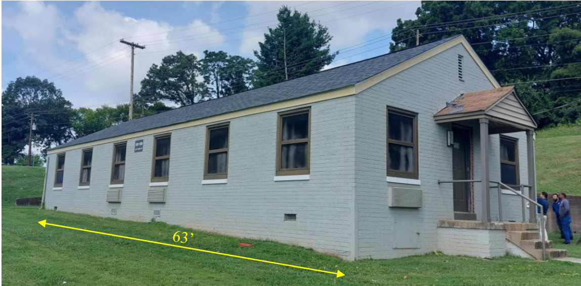
Figure 1. Duplex building at Western Heights, Knoxville, TN to be retrofitted with composite cladding panels as a first phase.
