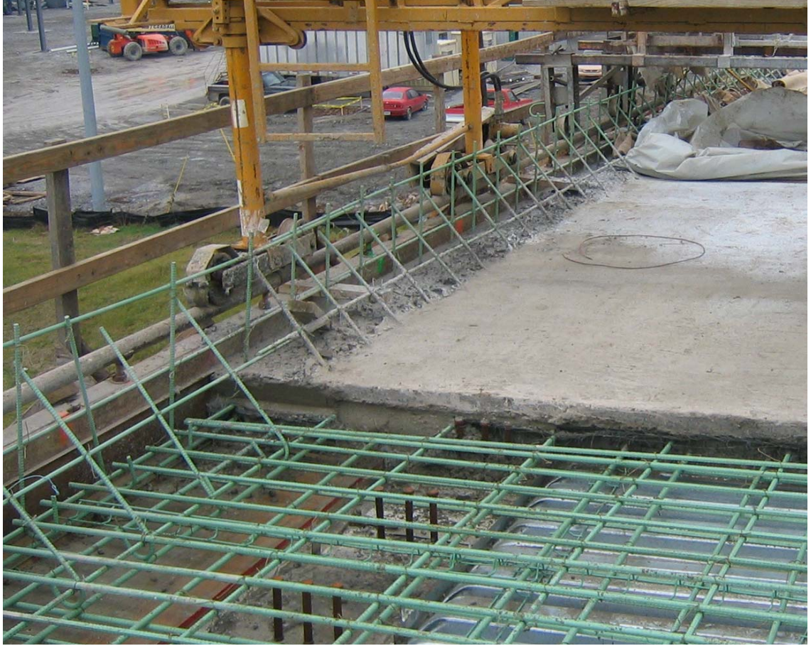
Figure 26: Typical scene at the start of the 2 nd day of the deck pour of the Massman Drive Bridge. Note that no attempt has been made to finish or smooth the surface of the deck that that is enclosed between the “J” shaped reinforcing bars (B 471E bars) protruding from the deck.
