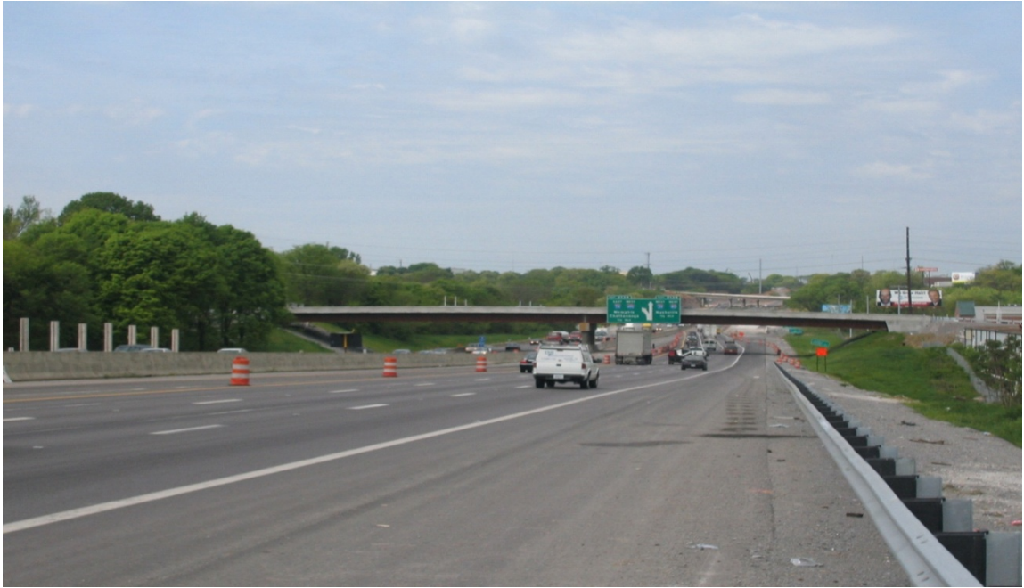
Figure 11: Photograph of Massman Drive Bridge Elevation Looking West.
