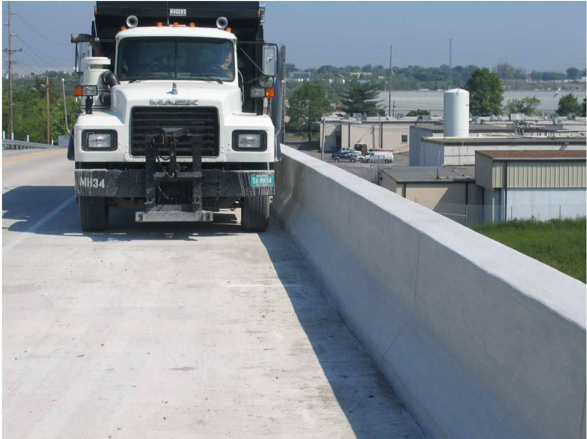
Figure 24: Typical scene (looking North) during 2 nd controlled load test showing the parapet on the East side of the Massman Drive Bridge. Note the sawed joint in the parapet in the right foreground of the figure.
