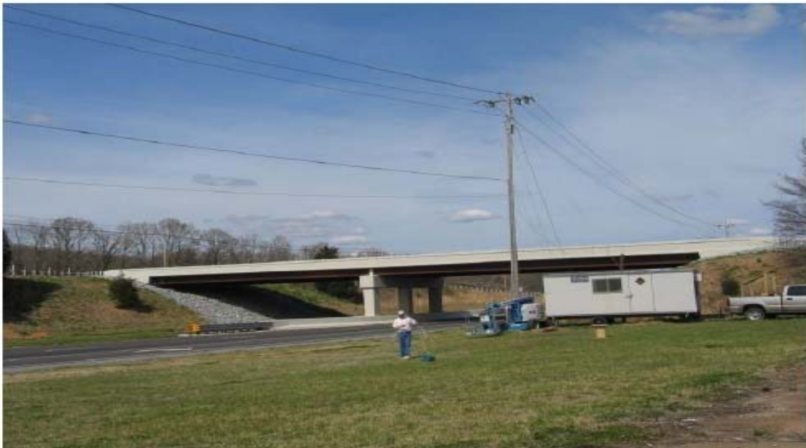
Figure 10: Photograph of DuPont Access Bridge Elevation Looking East.
