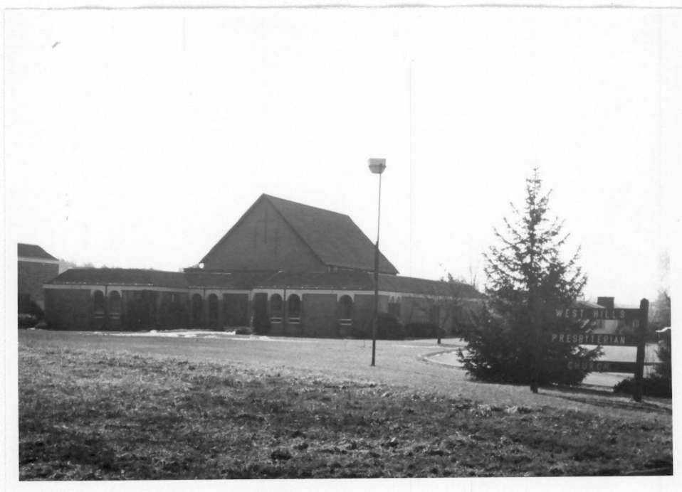
Figure 8. West Hills Presbyterian Church.
