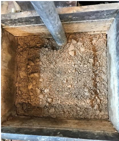
(c) Material B compaction
