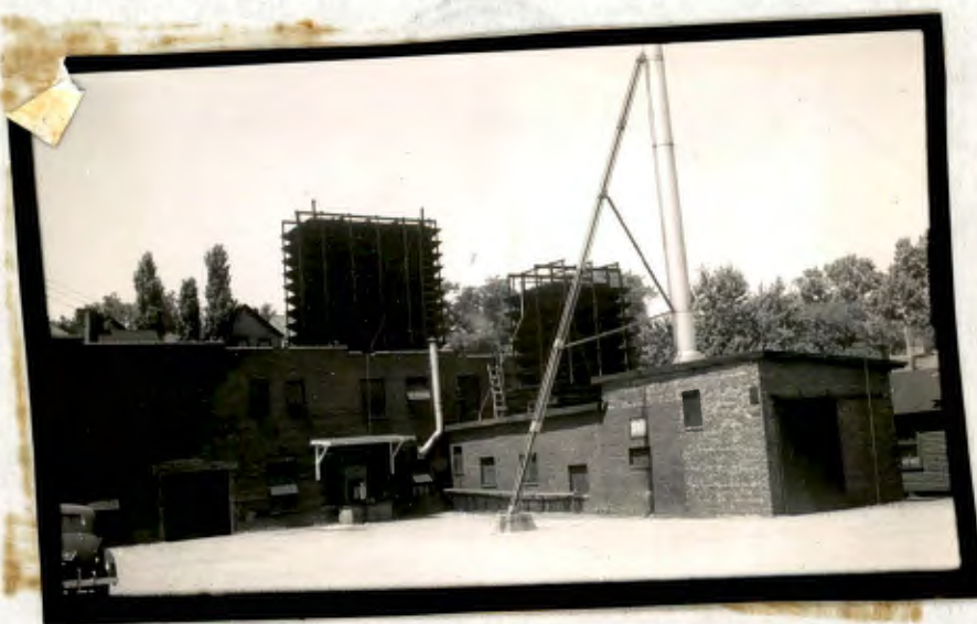
Side View - showing entrance to plant in the basement.
