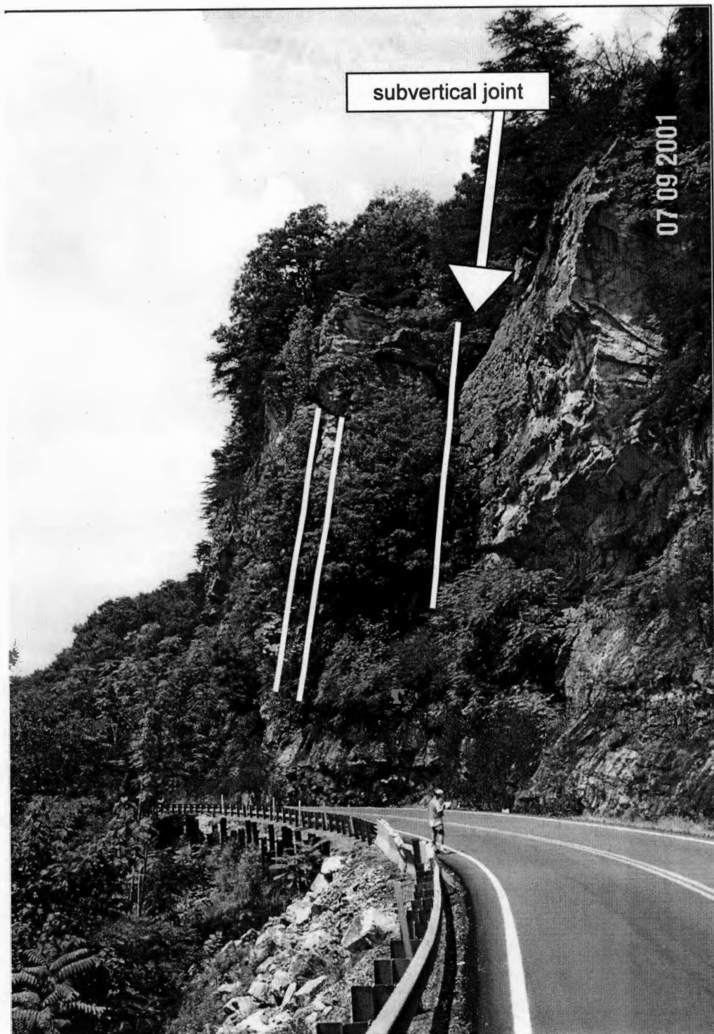
FIGURE 4. Roadcut B4 on Tennessee SR 30 showing large rock mass separating from slope face primarily along particular subvertical joint (arrow). View is to south.
