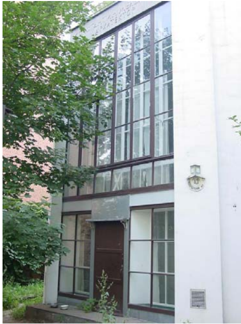
Fig. 6.4: Exterior of Melnikov House Source: Webshots, Inc
