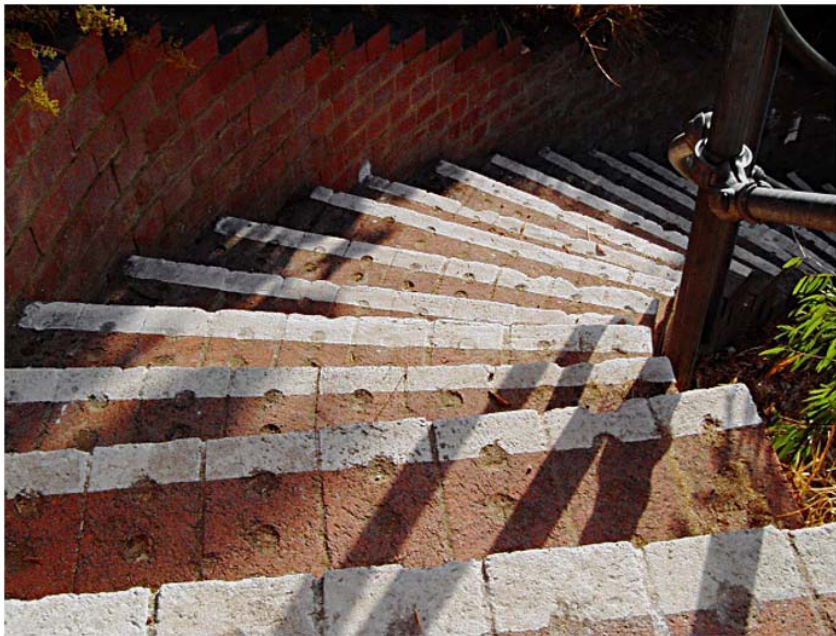
Fig. 2.4: Brick Stairway Source: Challenging Technologies, LLC
